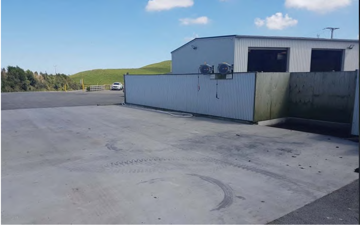
Photo 3 Truck wash area
