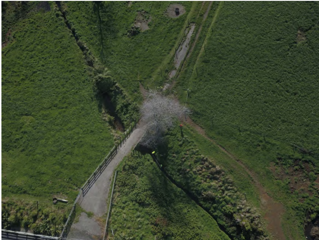
Photo 4 Aerial view of the wetland enhancement area (June 2022).
