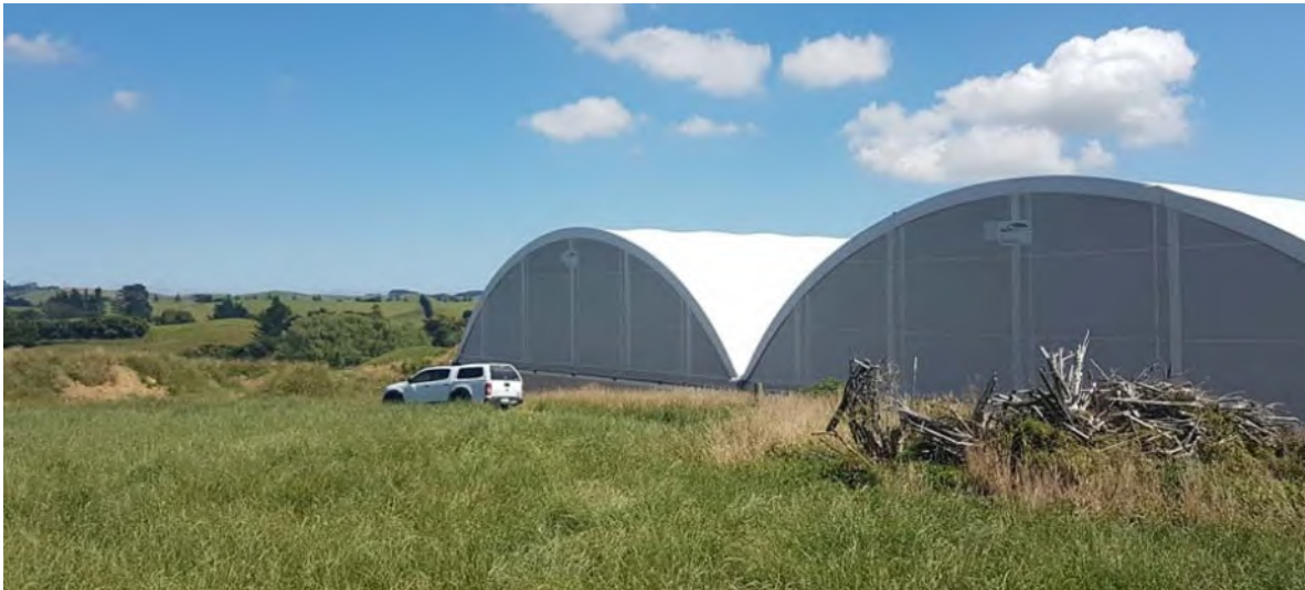
Photo 2 Rear of the Osflo main storage facility
