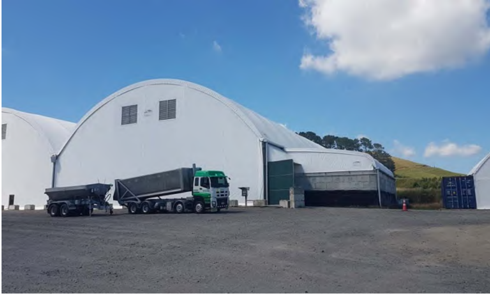
Photo 1 Osflo facility main storage facility
