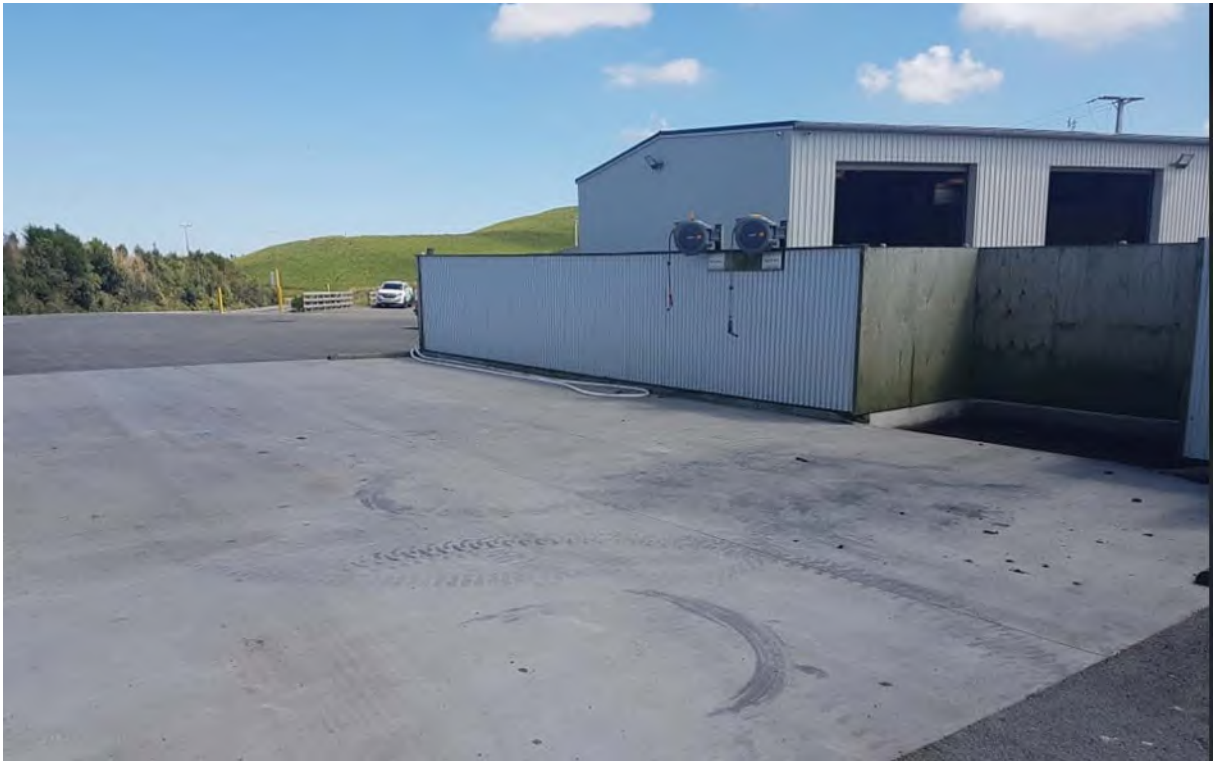
Photo 3 Truck wash area
