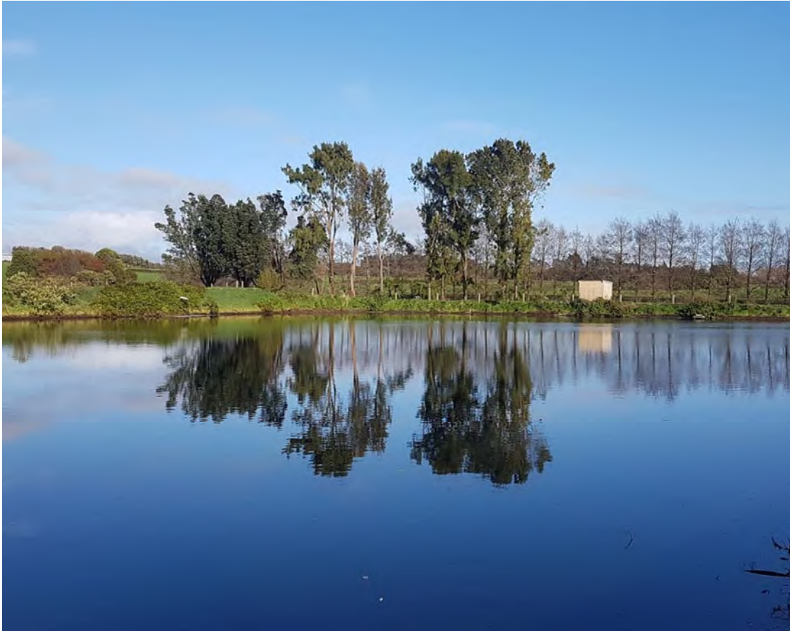
Figure 9 Pump shed on the final aerobic pond for spray irrigating treated piggery effluent to land
