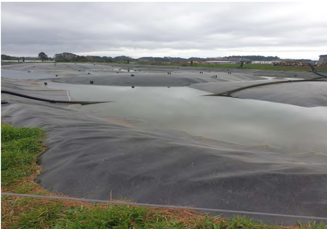
Figure 10 Covered anaerobic digester pond capturing methane for power production
