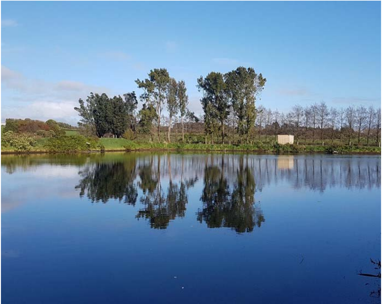
Figure 11 Pump shed on the final aerobic pond for spray irrigating treated piggery effluent to land
