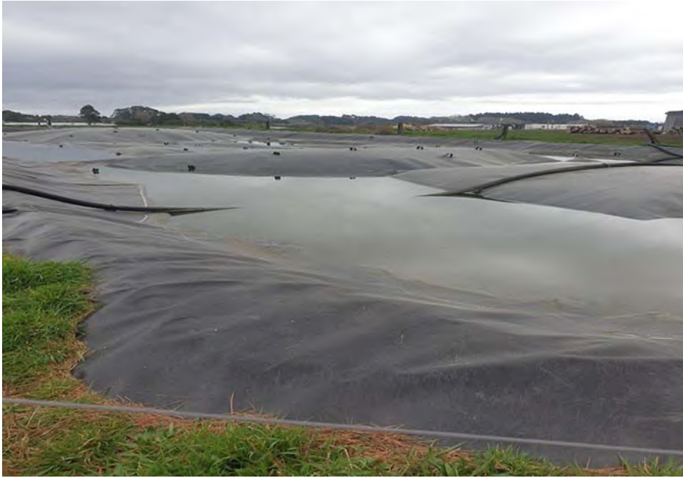
Figure 12 Covered anaerobic digester pond capturing methane for power production
