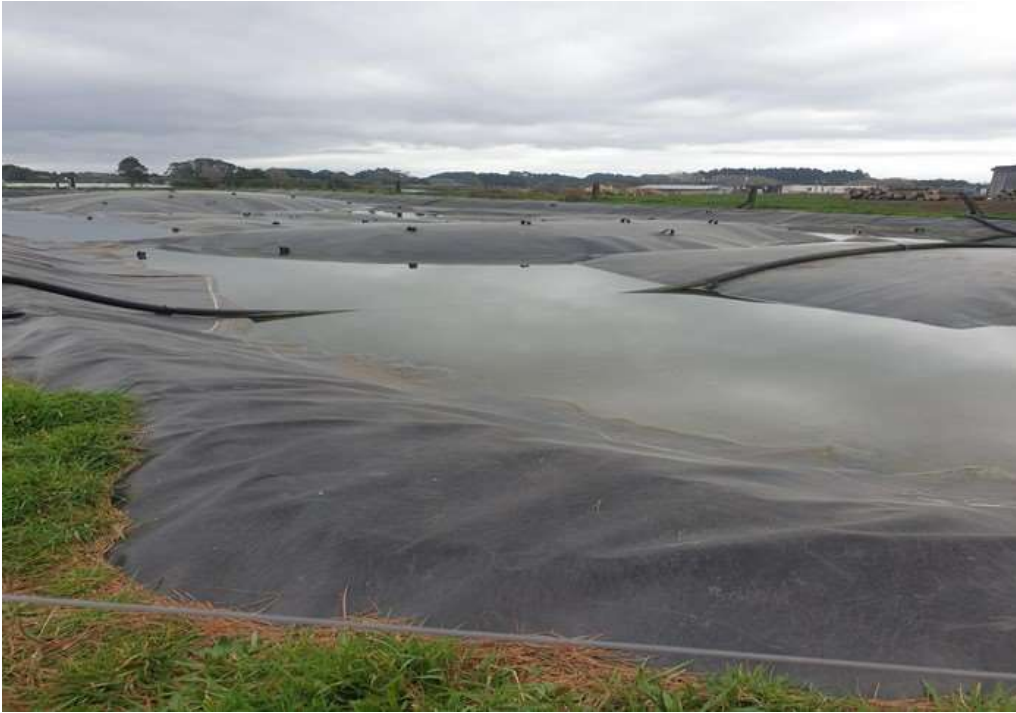
Photo 2 Covered anaerobic digester pond capturing methane for power production
