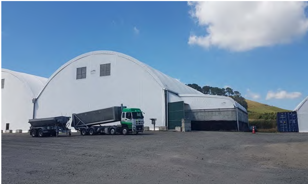
Photo 1 Osflo main storage facility
