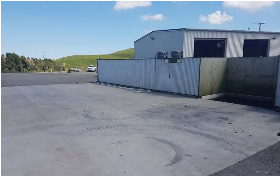
Photo 3 Truck wash area
