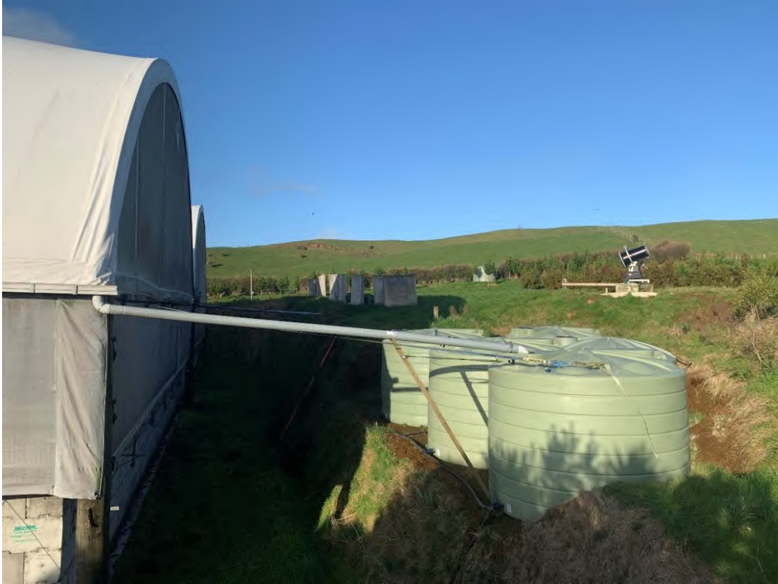
Photo 2 Rear of the Osflo main storage facility (2024)
