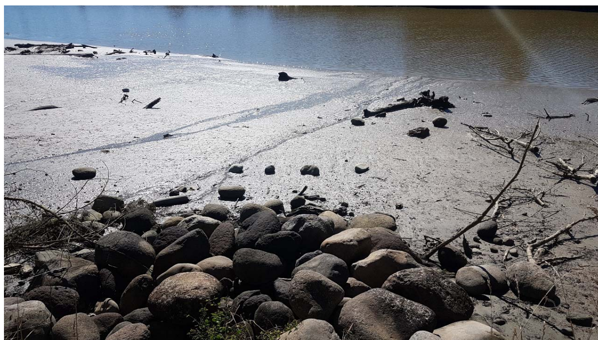
Photo 8 View of the discharge point from the Patea WWTP emergency overflow structure, February 2018
