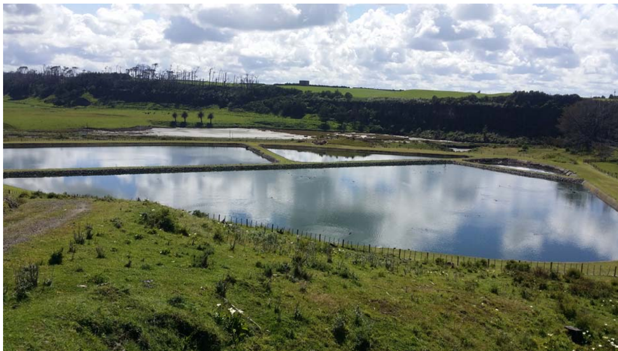
Photo 6 View of Patea WWTP
