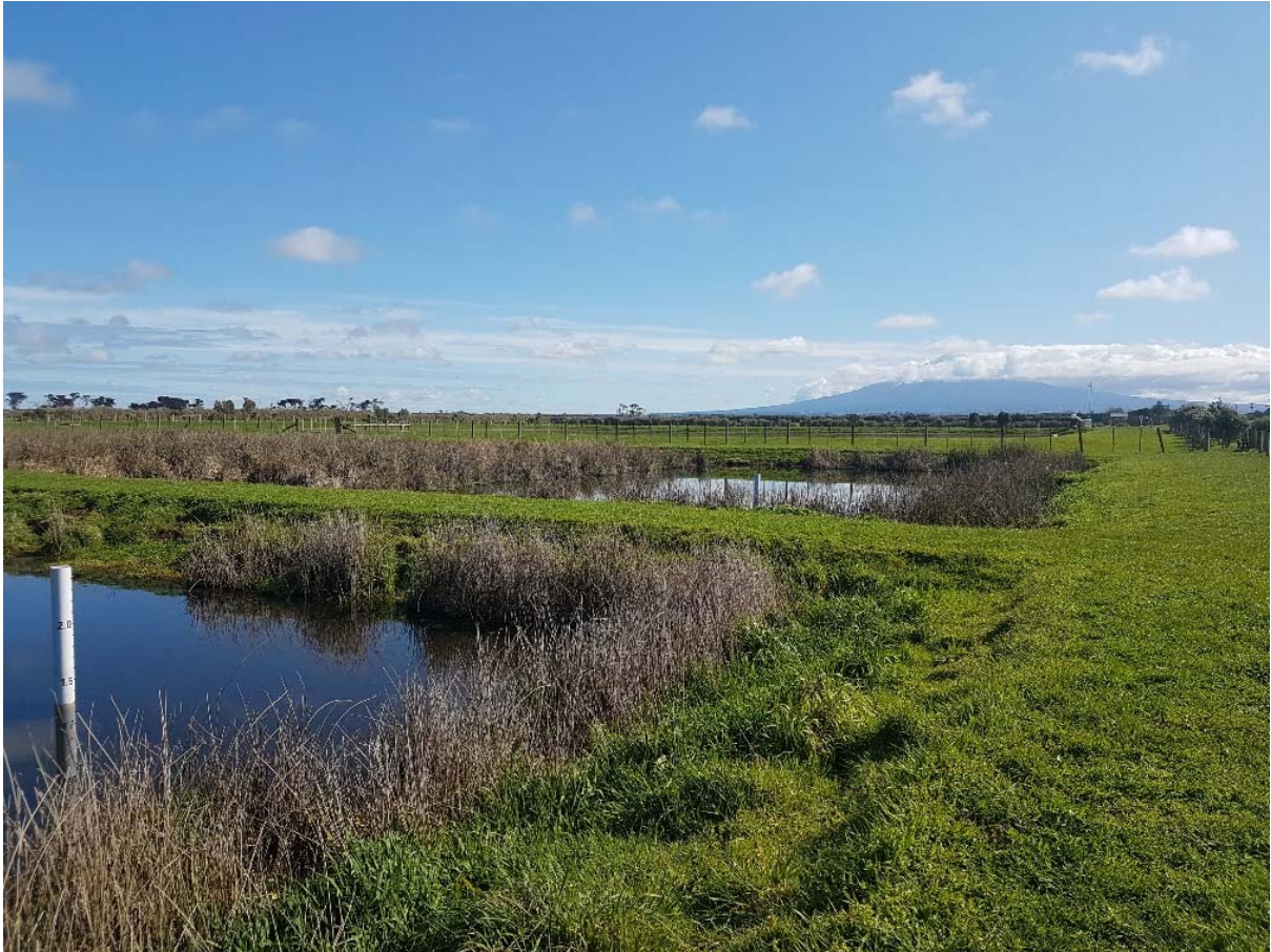
Photo 3 Manaia WWTP showing view of wetlands
