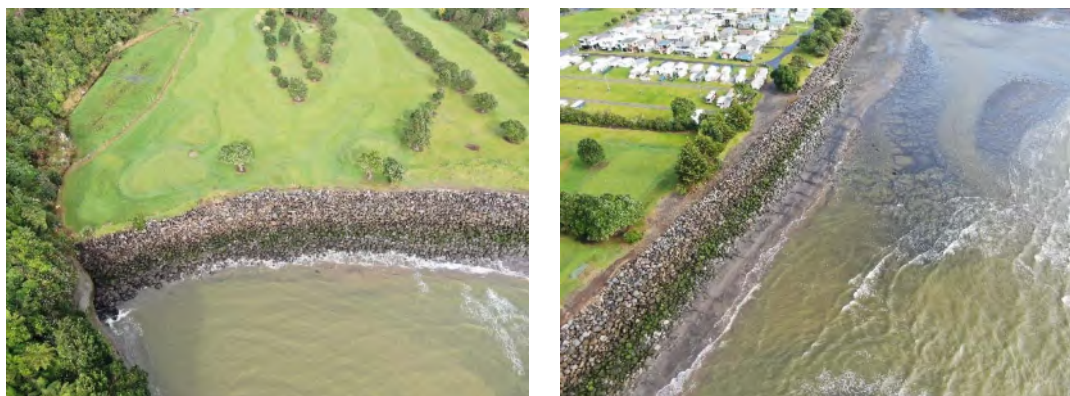
Photo 4 Urenui Beach rock rip rap seawall, June 2021
