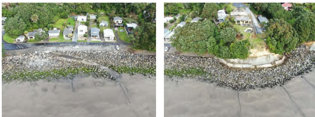
Photo 5 Onaero Beach rock rip rap seawall, June 2021
