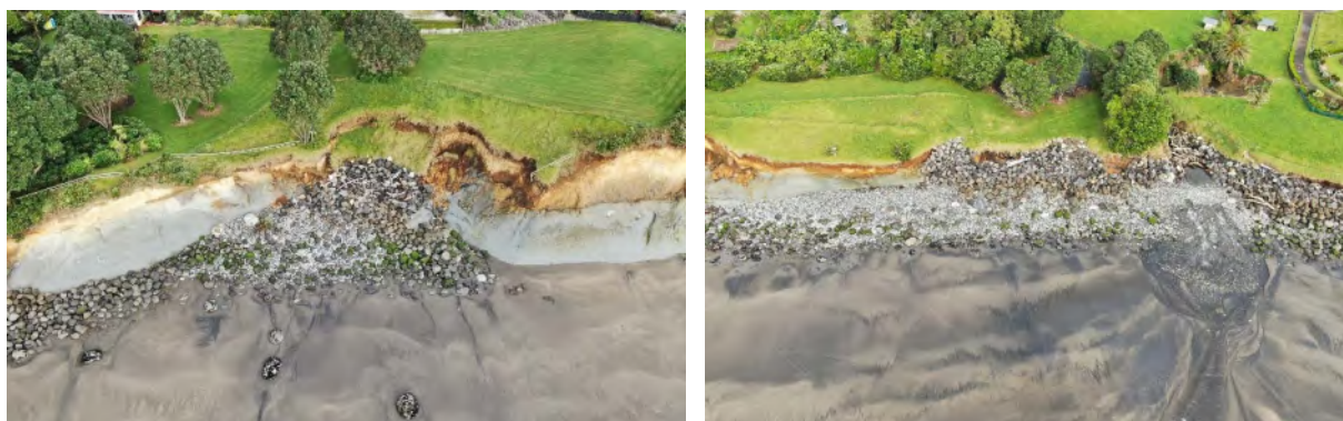
Photo 6 Onaero Beach rock rip rap incision repairs, June 2021
