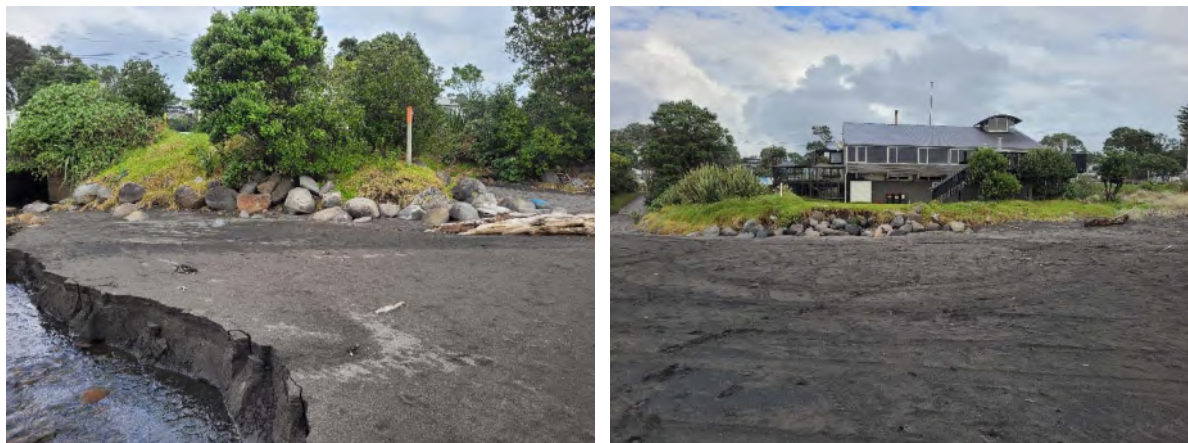
Photo 3 Oakura Beach rock protection structures 5523 (left) and 4584 (right), 8 June 2022
