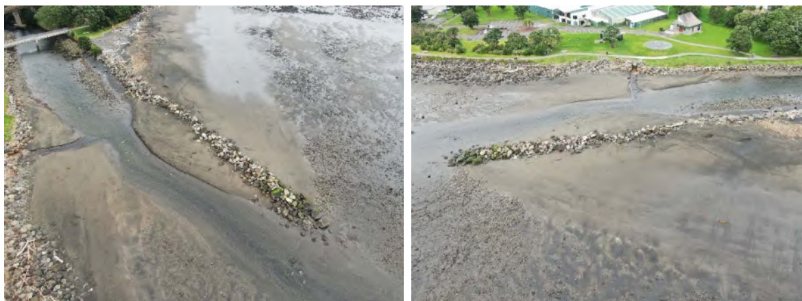
Photo 10 Te Henui rock rip rap groyne, June 2021
