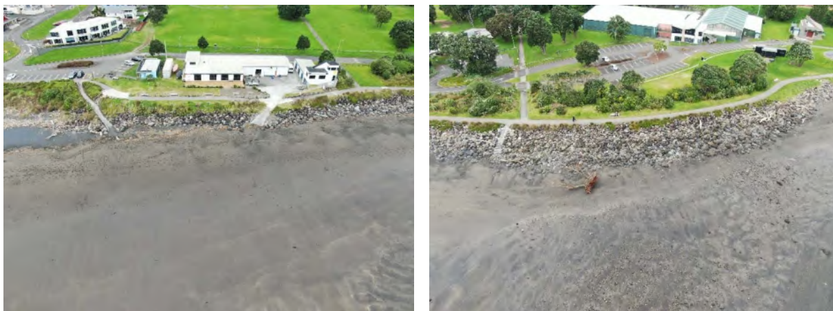
Photo 9 East End rock rip rap seawall, June 2021
