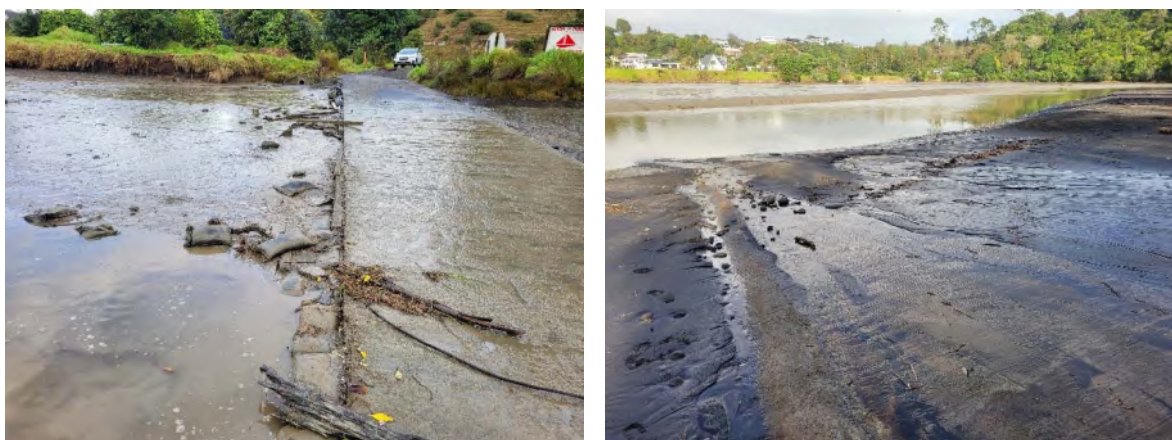
Photo 2 Displaced sand bags at the Tongaporutu boat ramp (left), and sand deposition on the Urenui boat ramp (right), 8 June 2022
