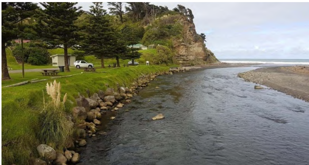
Photo 3 Looking downstream along rock protection works in the Kaupokonui Stream (April 2017)
