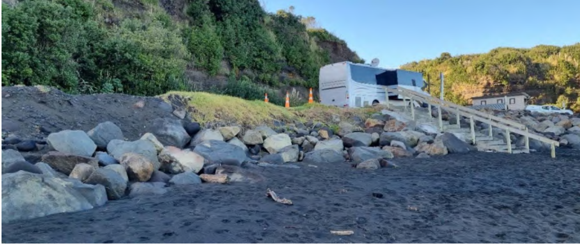
Photo 10 Northern end of Middleton Bay seawall (13 June 2023)
