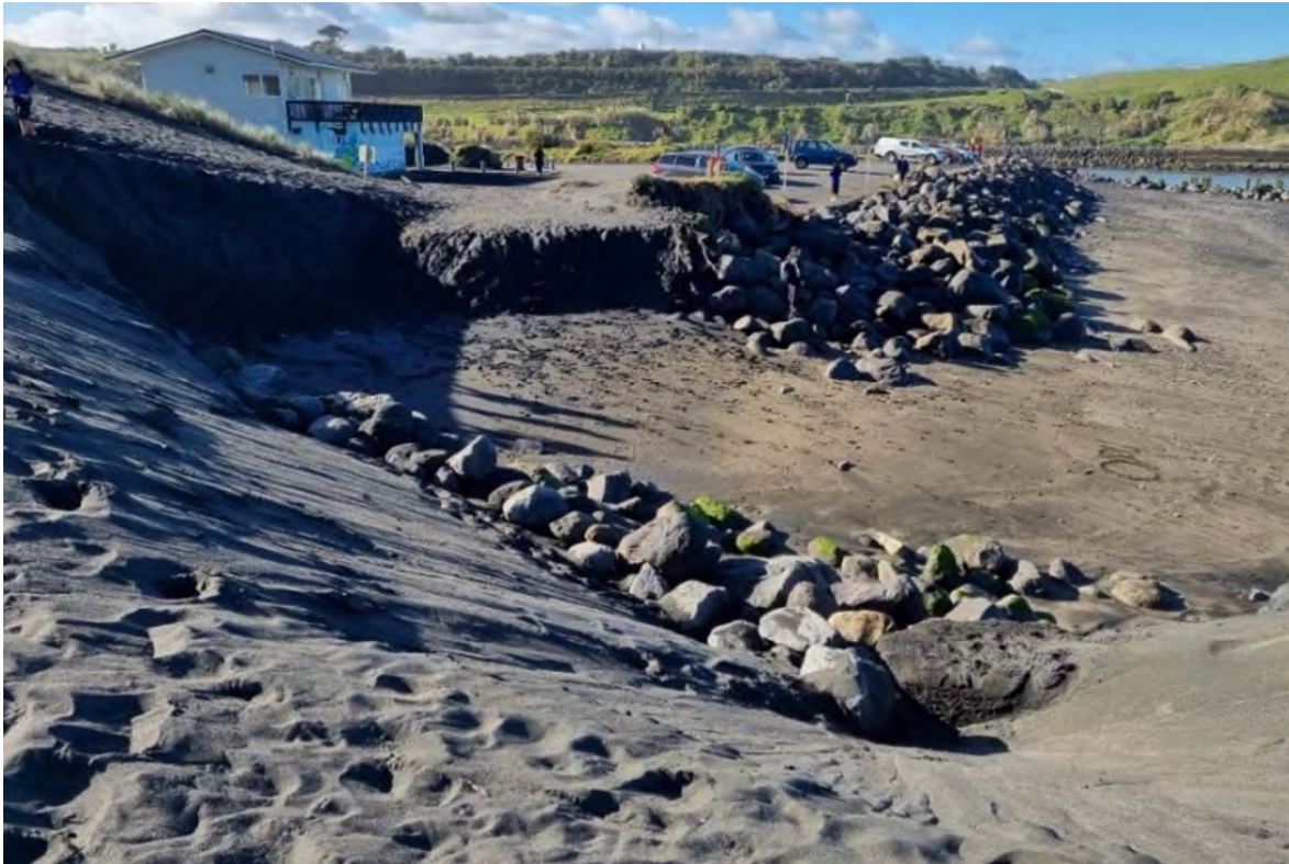
Photo 14 Eroded access from carpark to Pātea beach (13 June 2023)
