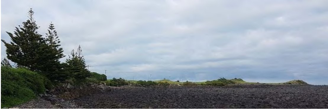
Photo 1 Bayly Road seawall (April 2017)
