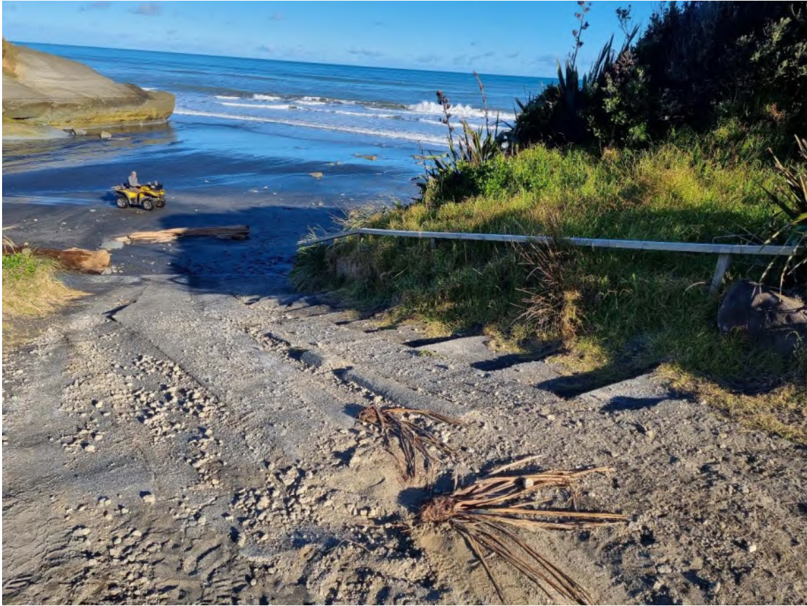
Photo 24 Caves Beach access ramp (13 June 2023)
