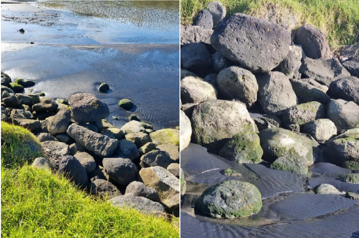
Photo 20 Perched rocks on rock wall downstream of boat ramp (13 June 2023)
