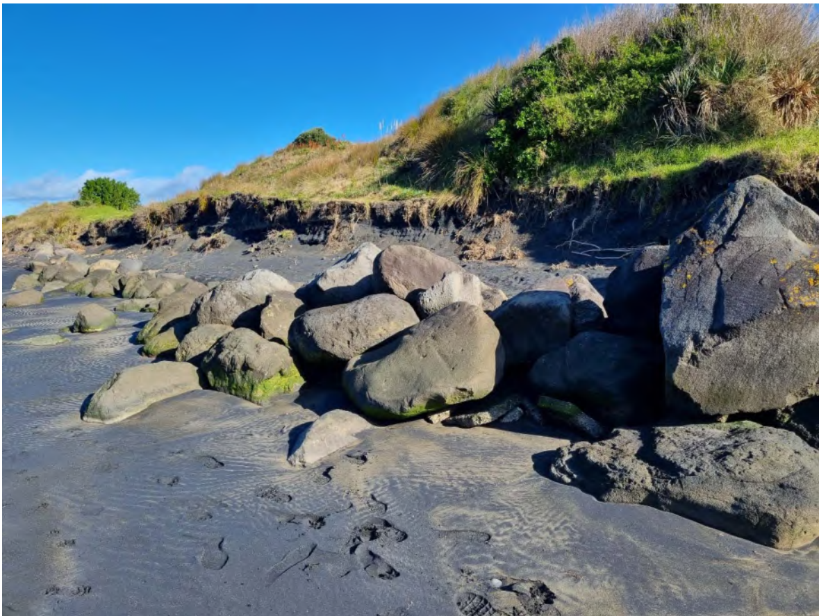
Photo 21 Erosion behind rock wall downstream of boat ramp (13 June 2023)
