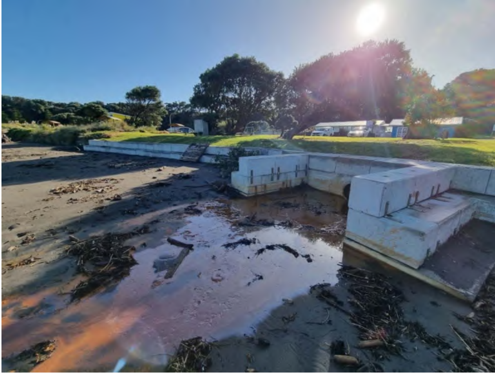
Photo 12 Opunake Beach replacement structure (13 June 2023)
