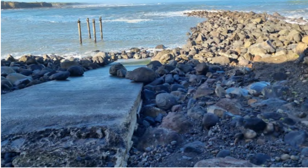
Photo 11 Ōpunake Bay boat ramp and rock groyne (13 June 2023).
