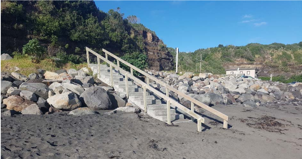
Photo 2 Middleton Bay seawall and staircase (9 June 2021)
