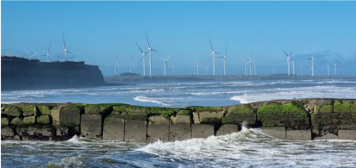
Photo 15 Southern mole slumping (13 June 2023)
