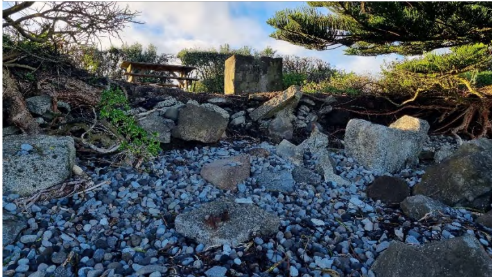
Photo 7 Section of Bayly Road seawall below picnic table and pine trees (13 June 2023)
