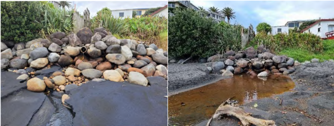
Photo 1 Beach level from June 2022 (left) compared to June 2024 (right) at the Messenger Terrace stormwater outfall
