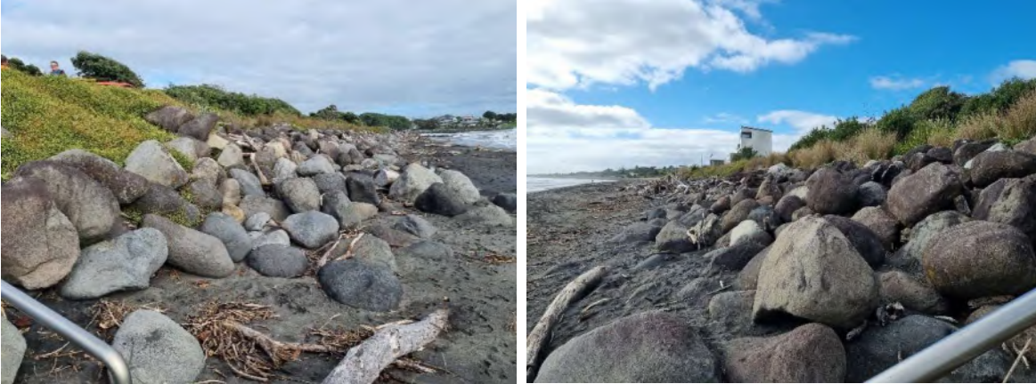
Photo 14 East End rock rip rap seawall, June 2021
