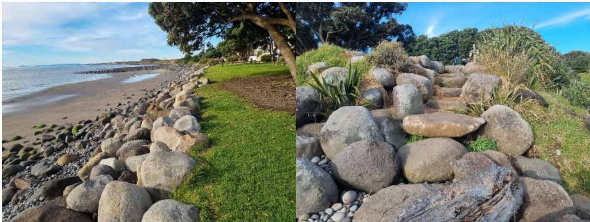
Photo 12 Bell Block rock wall and access, June 2024
