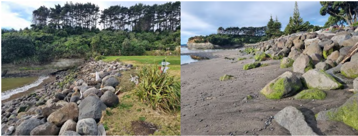
Photo 6 Urenui Beach rock rip rap seawall, June 2024
