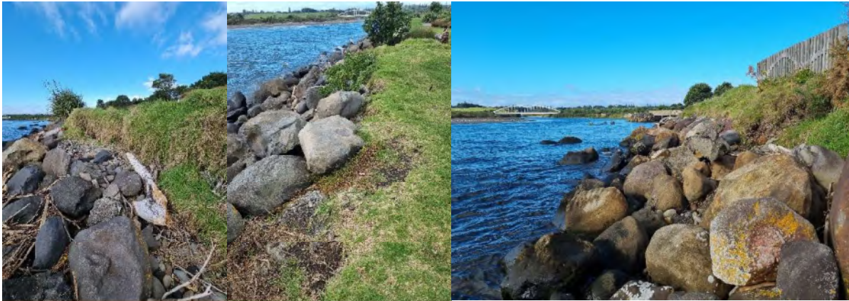
Photo 3 Waiwhakaiho riverbank protection, June 2024
