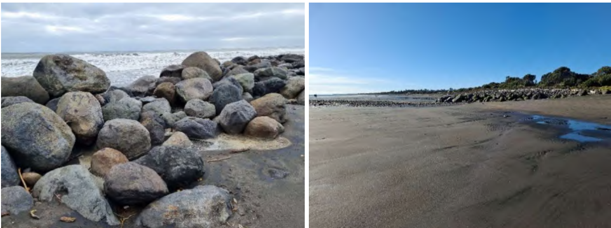
Photo 15 Te Henui rock rip rap groyne, June 2024
