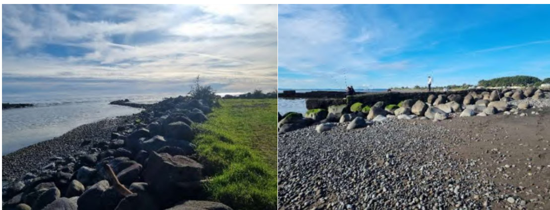
Photo 9 Waitara River mouth training wall structures, June 2024
