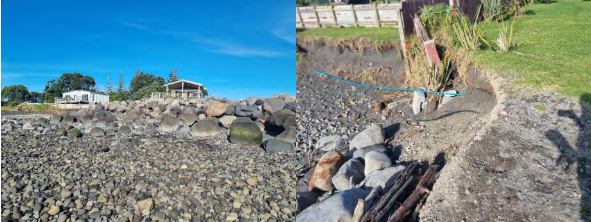
Photo 10 Area of recent works with added rocks (left) and adjacent area of recent erosion (right) in Waitara, June 2024
