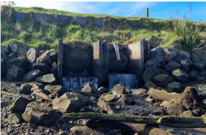
Photo 5 Waitara outlet structure 7718-1, June 2024
