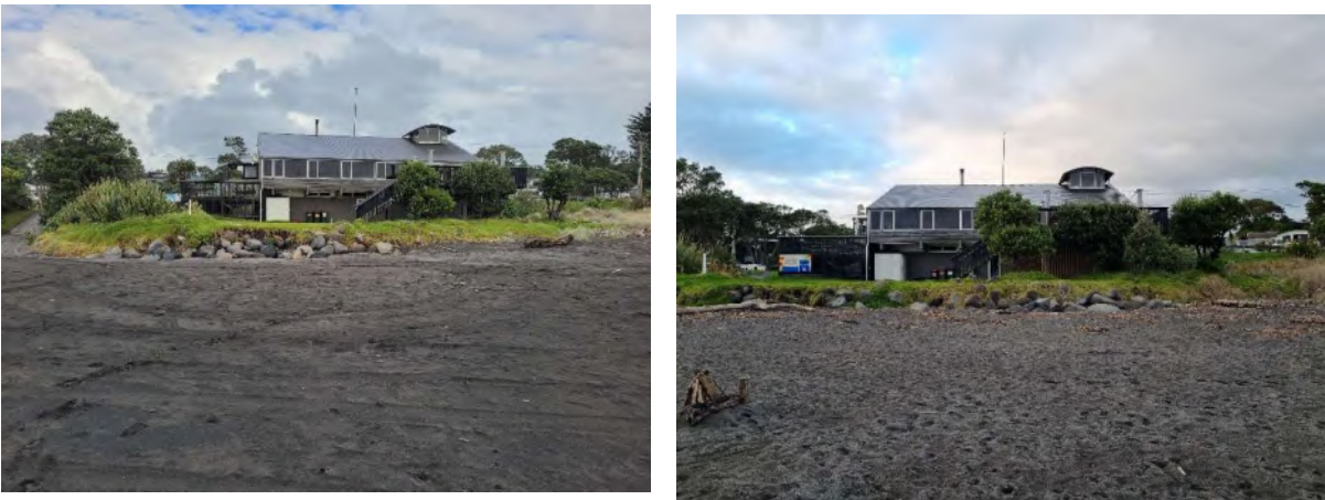
Photo 4 Oakura Beach rock protection structure 4584, 8 June 2022 (left); 11 June 2024 (right)
