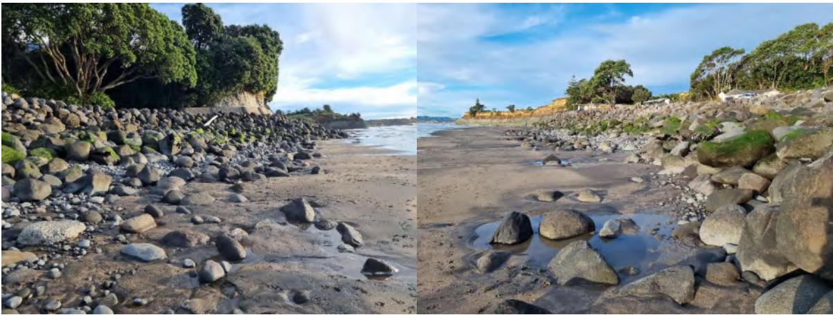
Photo 7 Onaero Beach rock rip rap seawall, June 2024
