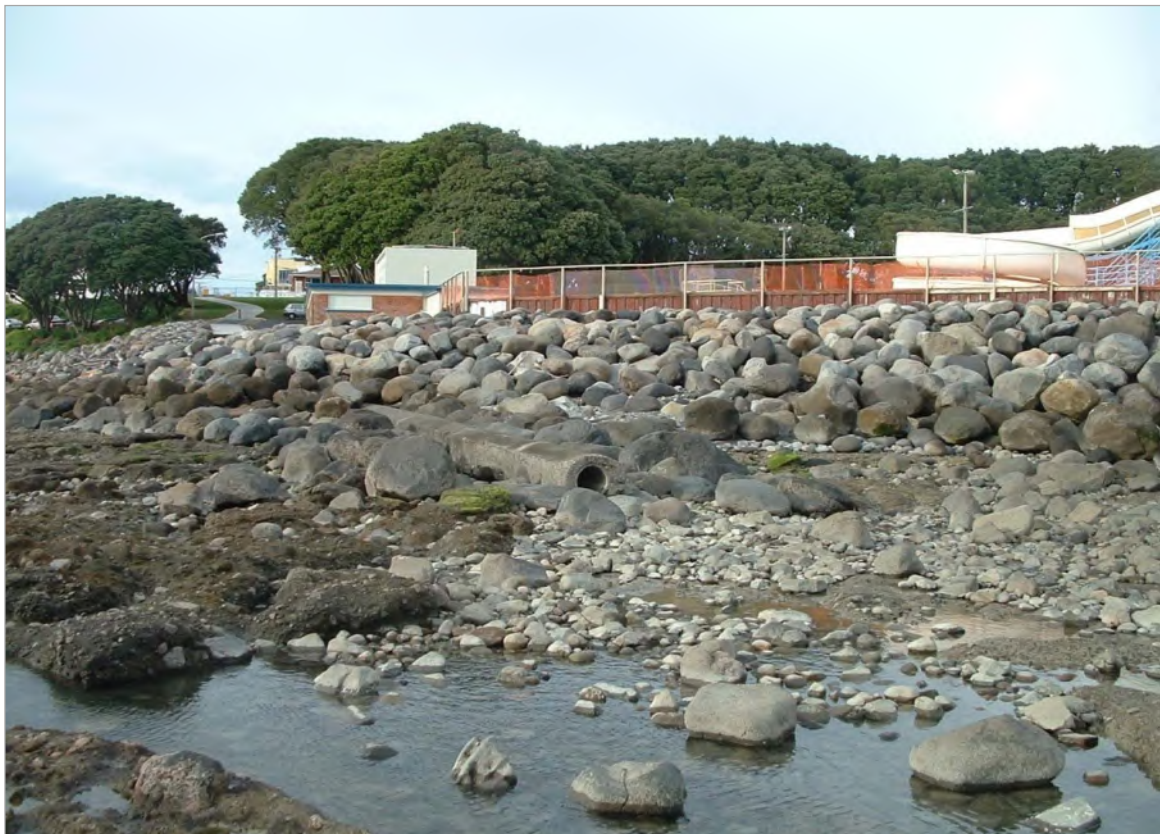
Photo 1 Aquatic Centre ocean outfall along the intertidal zone of the Kawaroa Reef
