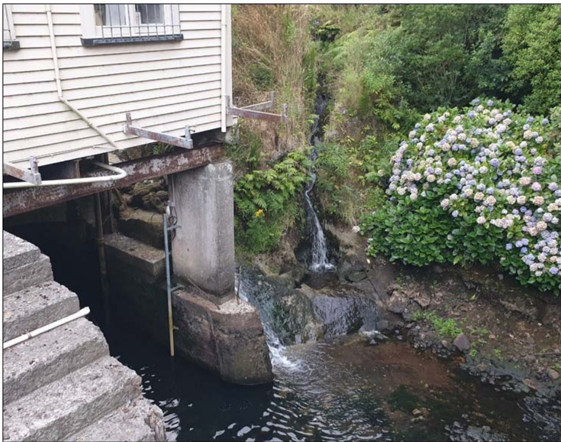
Photo 6 Two attractant flows that direct fish away from the trap. One small tributary (right) and one coming from the station (left beside the concrete pillar). There is a third residual flow from the station outlet pipe directly below the building (seen in Photo 7). Photo taken during the 2019 - 2020 monitoring period
