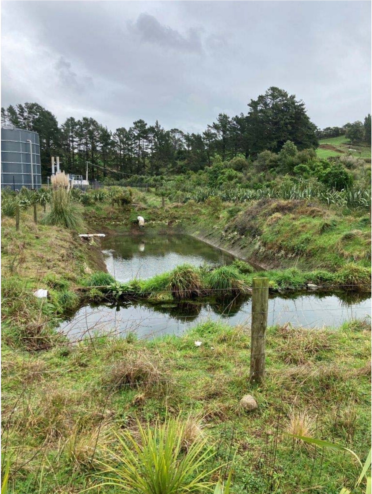
Photo 1 Stormwater sediment/retention ponds system
