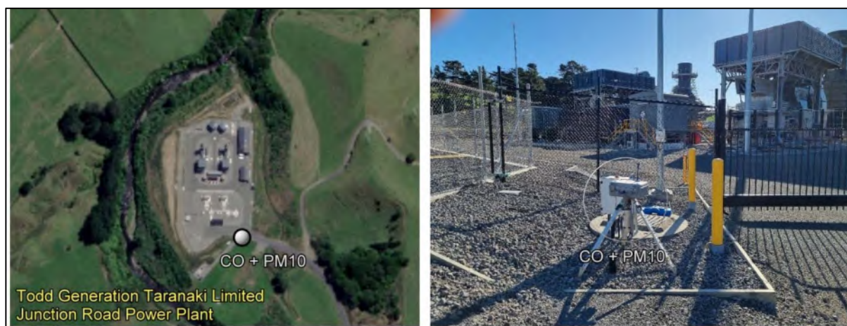
Figure 2 Air monitoring site at the Junction Road Power Plant (2021-2022)
