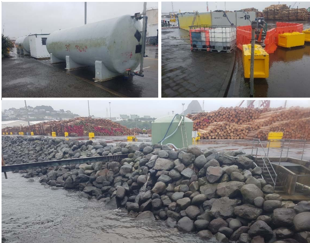
Photo 4 New stormwater containment and filtration units at outlet 32/STW001135 (top) and outlet 41/STW001157 (below)
