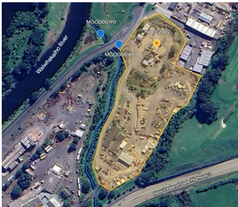
Figure 6 Aerial view of Downer site with associated sampling points
