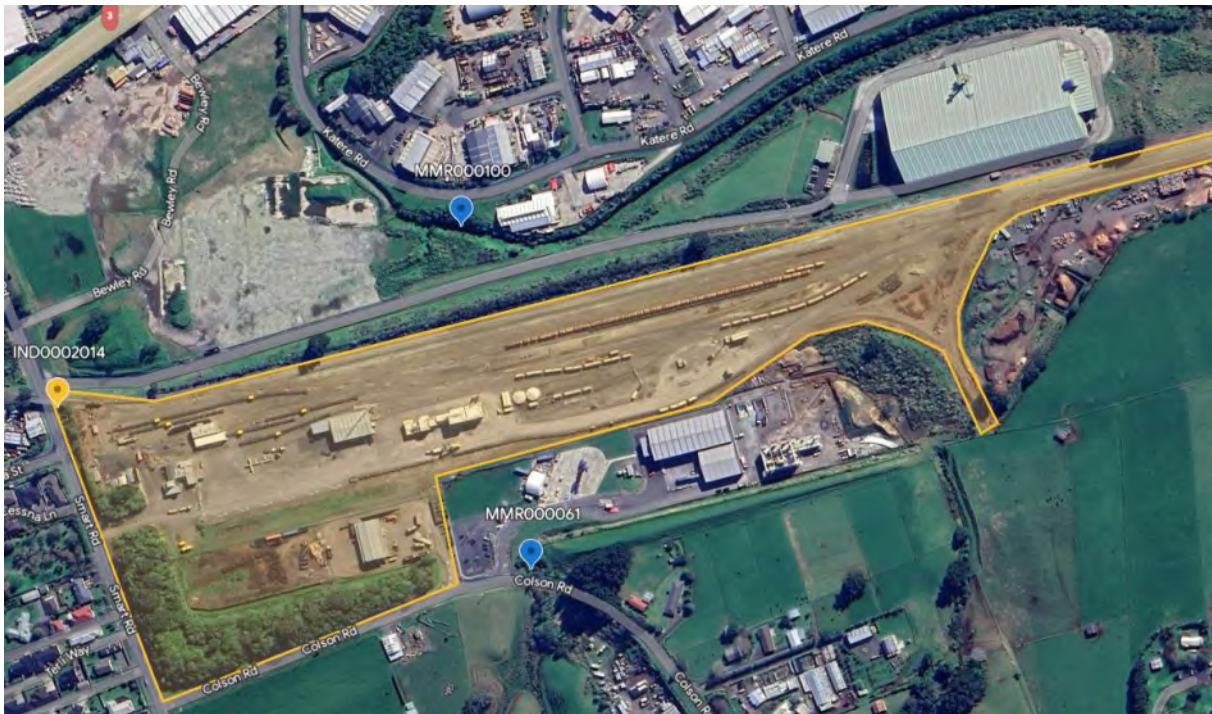
Figure 10 Aerial view of KiwiRail site with associated sampling points
