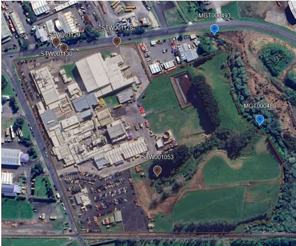
Figure 14 Tegel poultry processing plant site, with the location of the discharge sampling point
