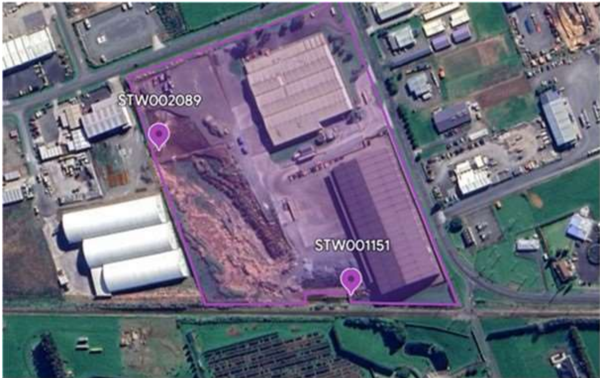
Figure 6 Aerial view of J Swap site, with the location of the associated discharge sampling points
