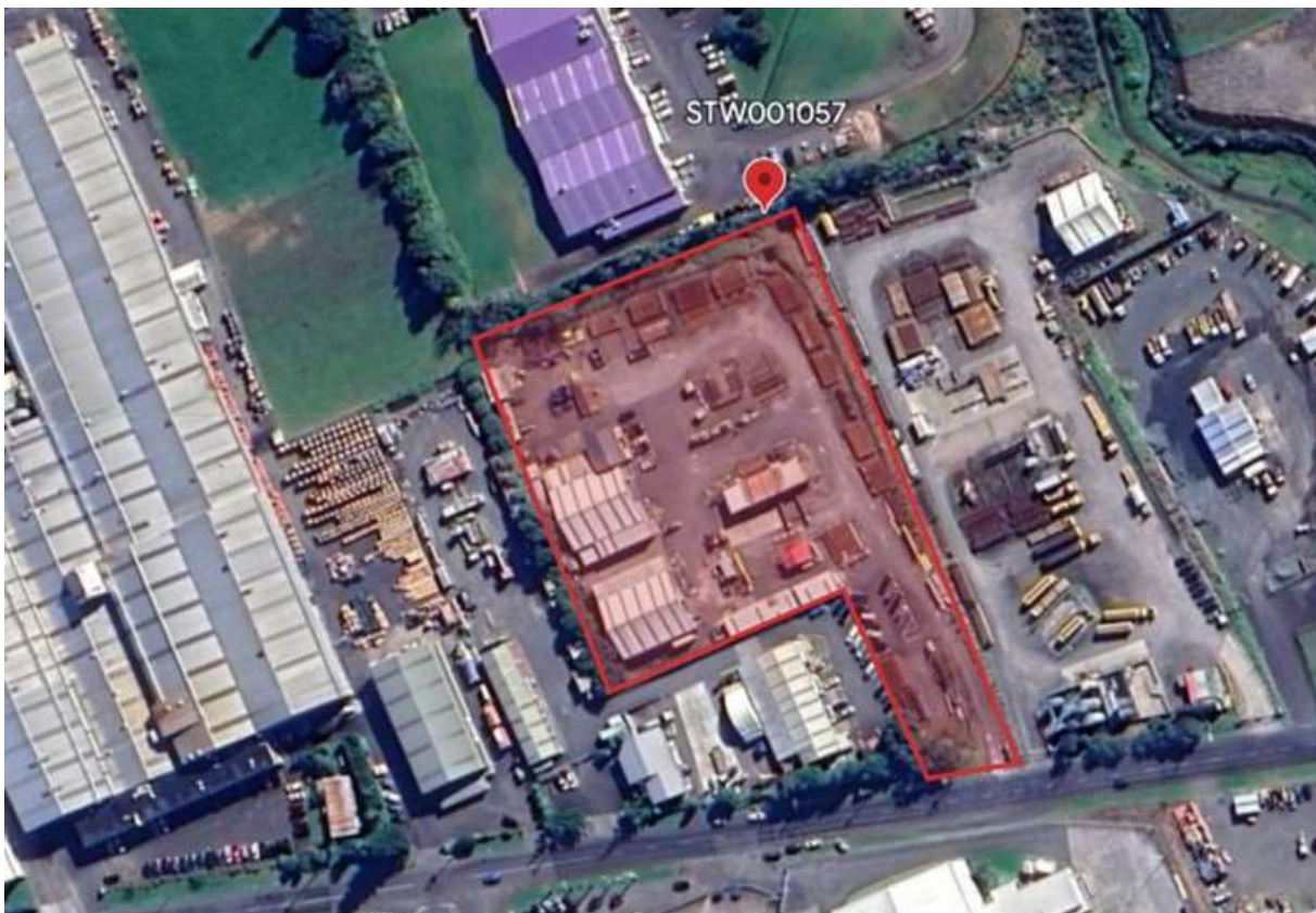
Figure 12 Aerial view of Tasman Tools site, with the location of the discharge sampling point
