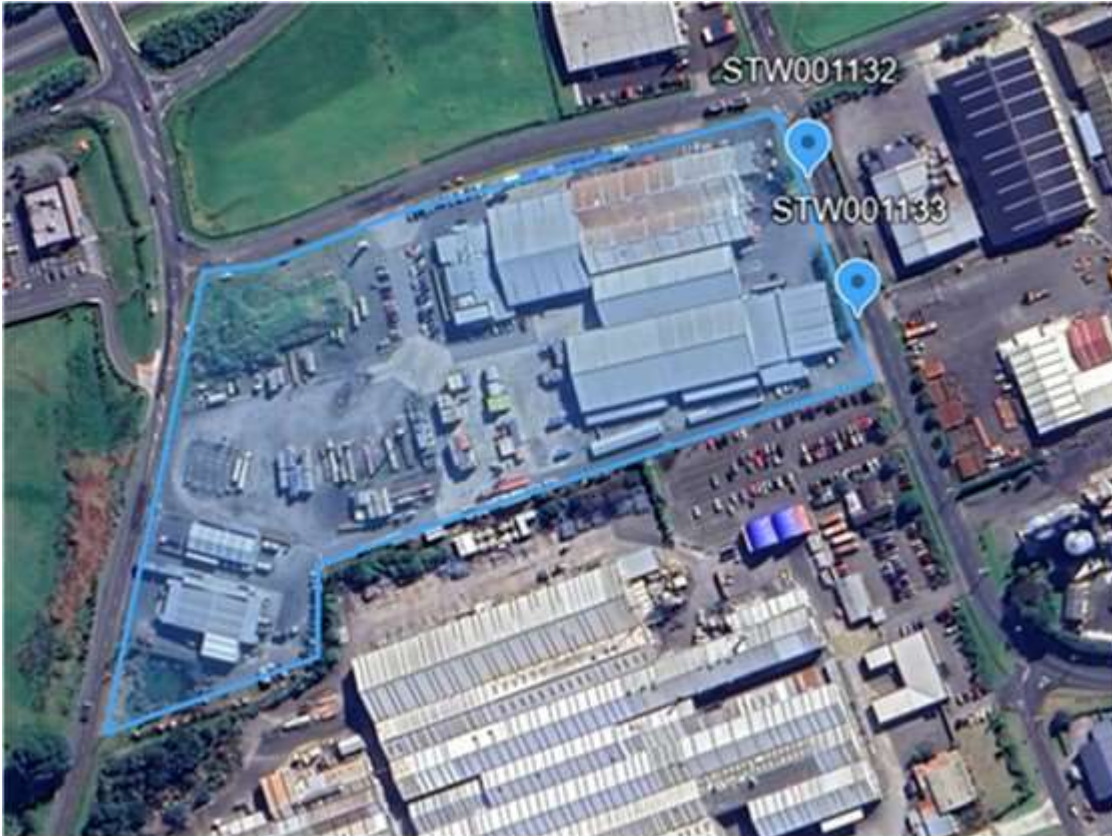
Figure 8 Aerial view of MOVE site, with the location of the associated sampling point
