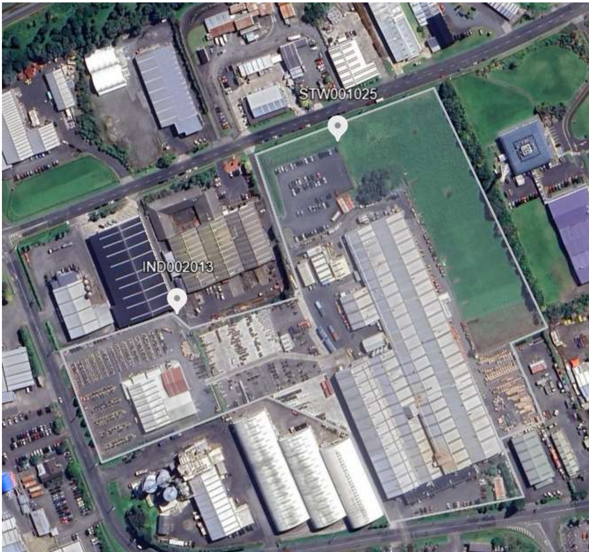
Figure 10 Aerial view of Nexans site, with the location of the sampling points
