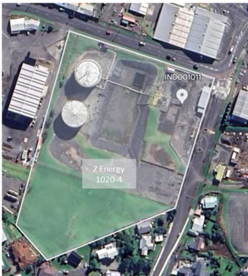
Figure 13 Aerial photograph of the Z Energy Ltd Ngamotu site and associated Taranaki Regional Council sampling point
