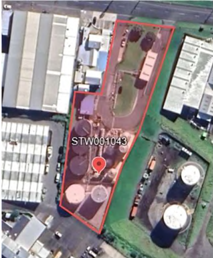
Figure 11 Aerial photograph of the Quantem site and associated Taranaki Regional Council sampling point
