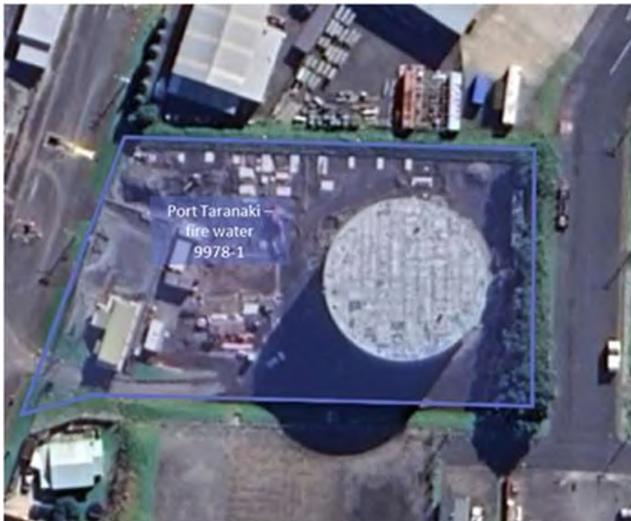
Figure 10 Aerial photograph of the Port Taranaki fire water storage facility
