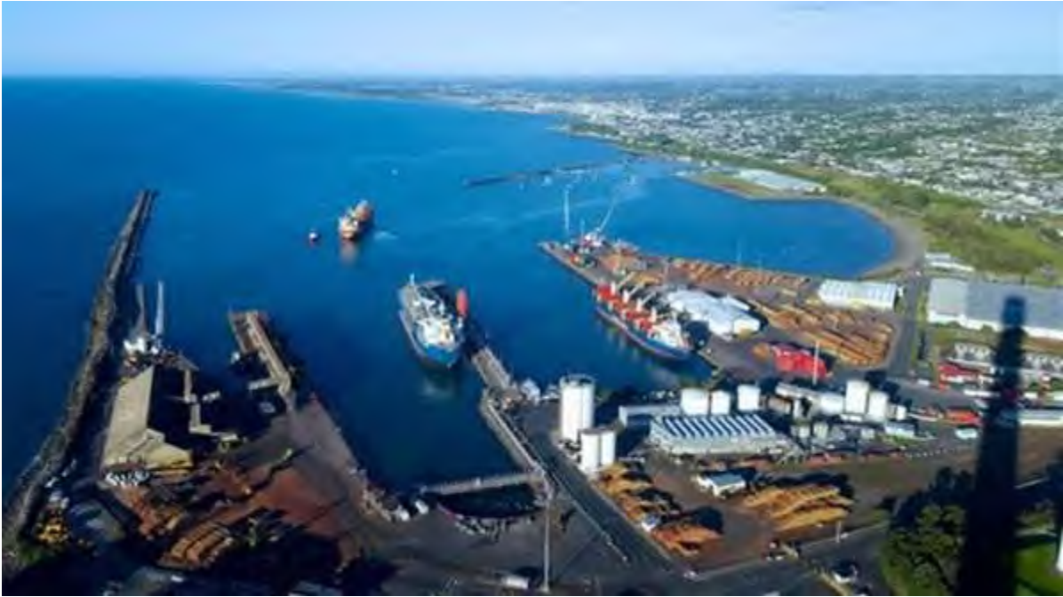
Photo 1 Port Taranaki industries from the chimney
