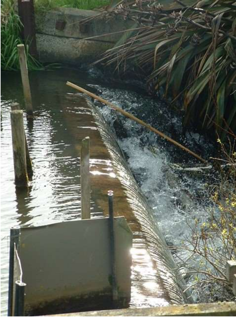
Photo 1 The weir and fish pass on the Tawhiti Stream (fish pass visible on far side)
