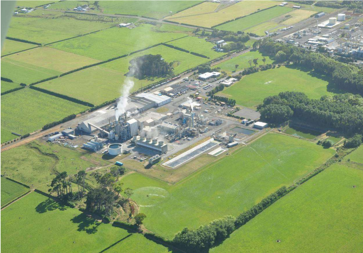
Photo 1 Ballance Agri-Nutrients ammonia urea plant (viewed looking towards the north-east)
