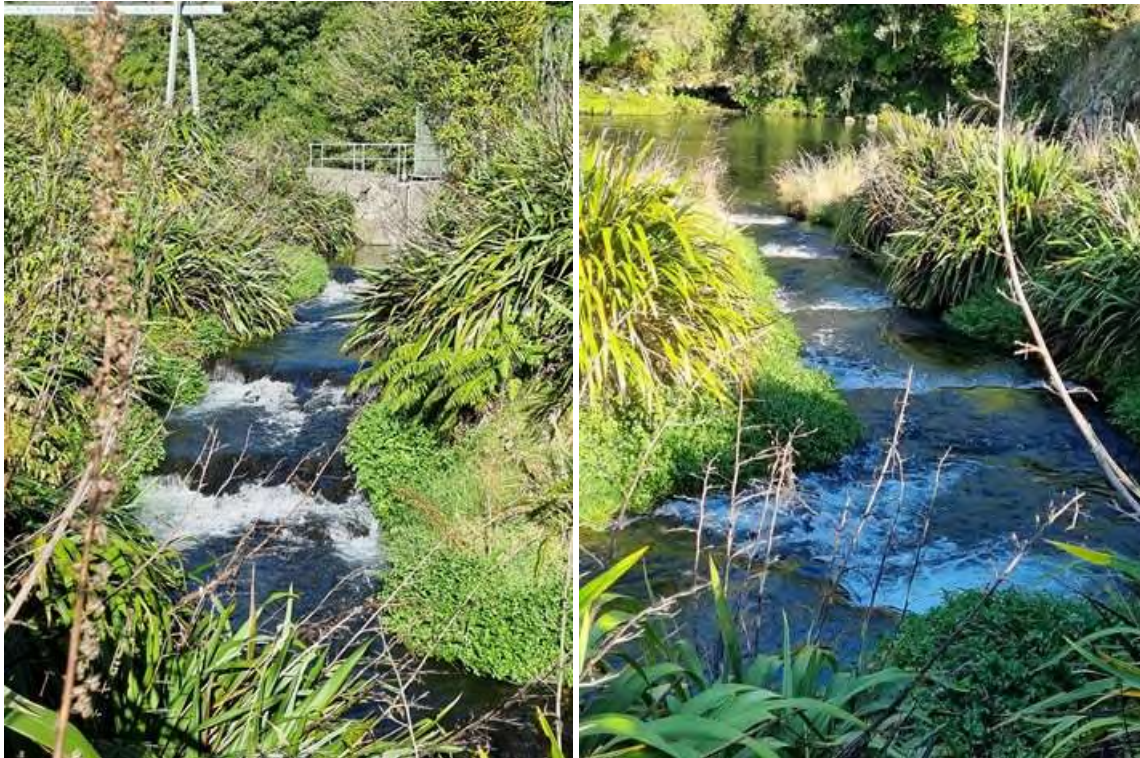
Photo 1 Photos of the fish pass, which has an approximate 90 degree bend midway
