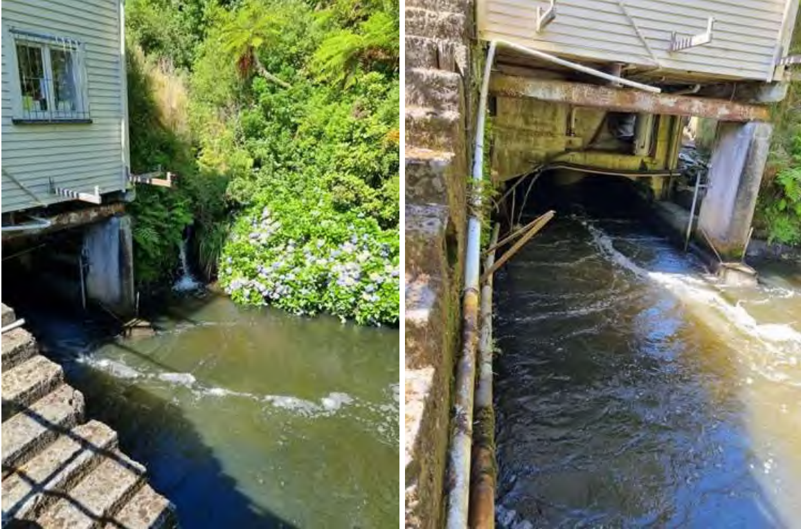
Photo 6 Left photo - Two attractant flows that direct fish away from the trap. One small tributary (right) and one coming from the station (beside the concrete pillar to the right (2023/24)). Right photo - there is a third residual flow from the station outlet pipe directly below the building (2023/24)
