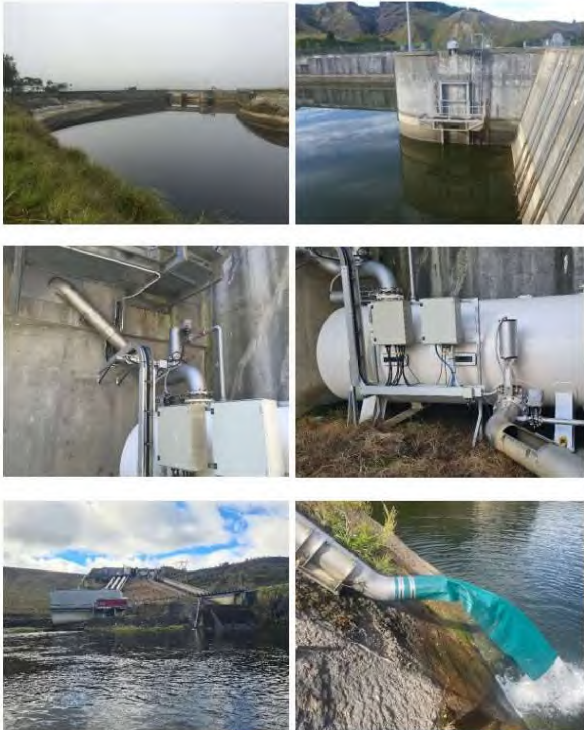
Figure 7 Pātea HEPS eel bypass system
