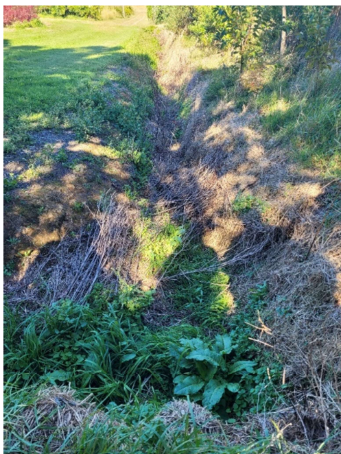
Figure 4 Farm drain on the neighbouring property
