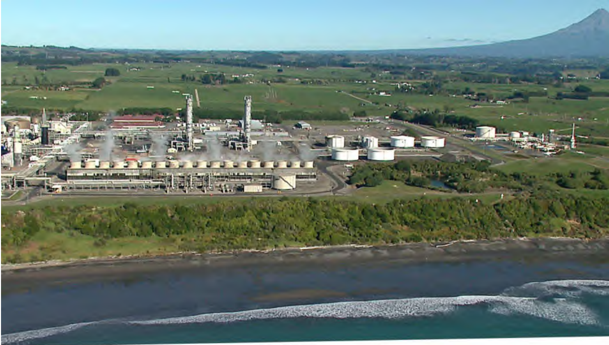
Photo 1 Cooling towers and distillation stacks at the Methanex Motunui site
