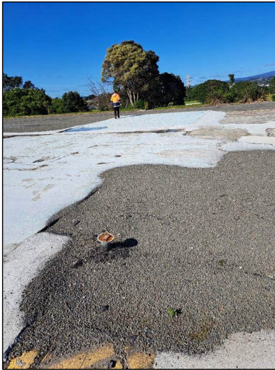
Photograph 1: Welded fill point for process water piping adjacent to Building 15.
