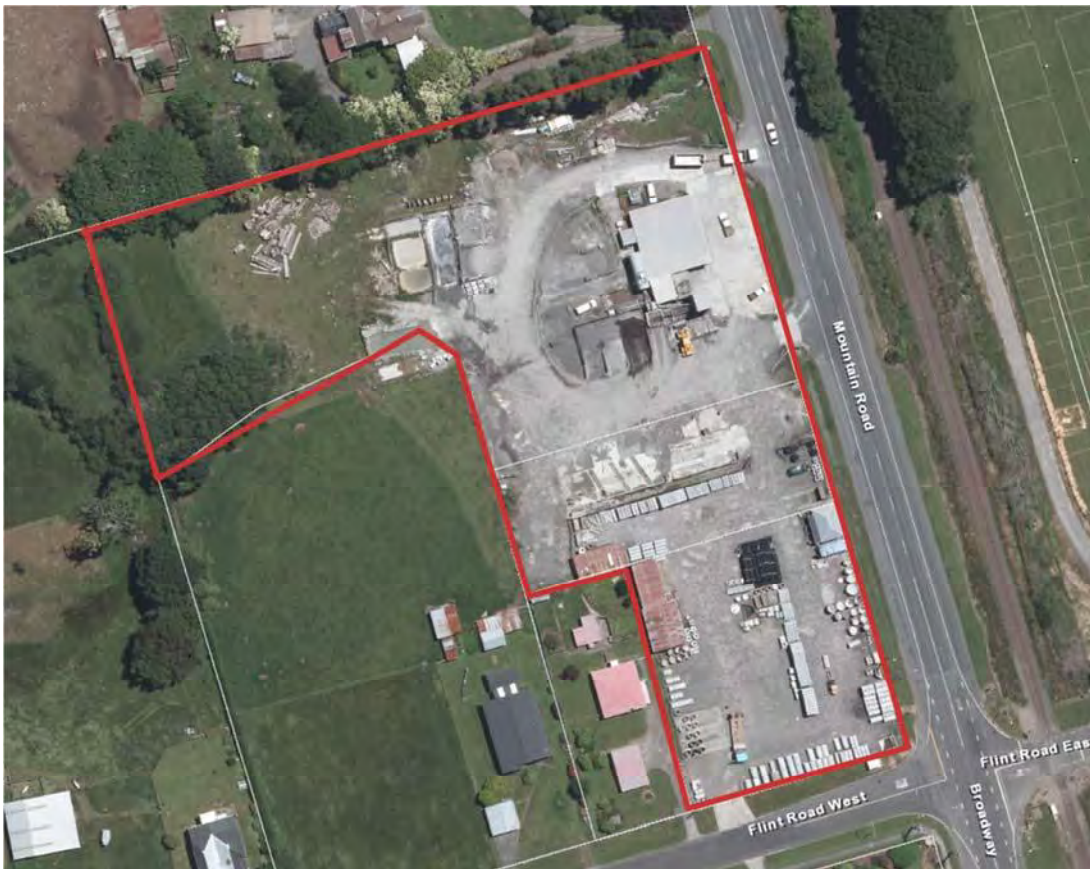
Figure 3 Fletcher Concrete site (Firth Industries and Humes Pipeline Systems), Stratford
