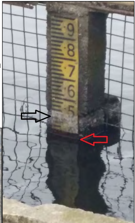
Photo 4 (right) The staff gauge at Opunake Lake, 2 October 2015. The black arrow marks the minimum lake level as per consent, the red arrow indicates the actual lake level.
