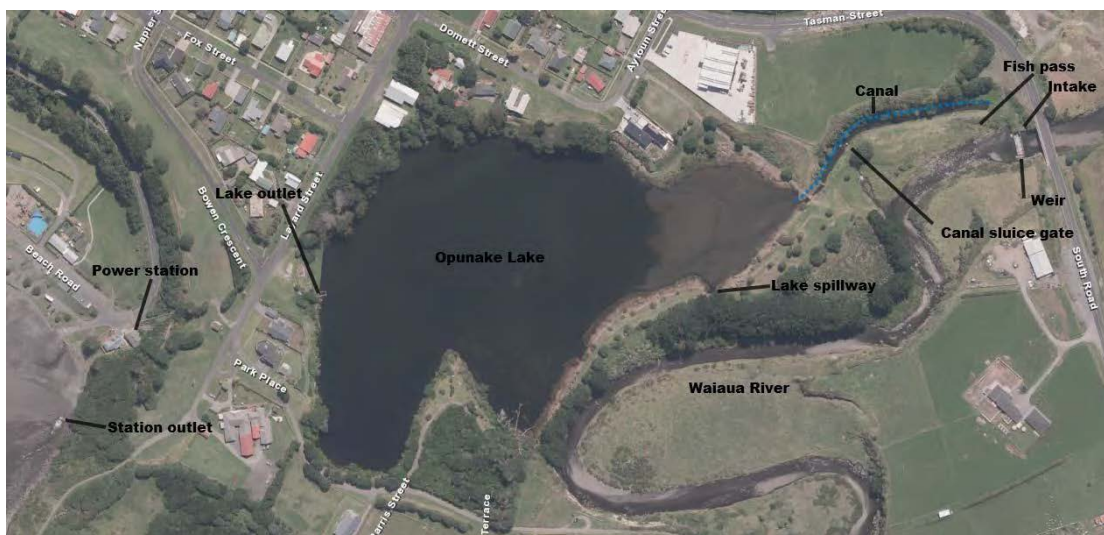
Photo 1 Opunake Hydro Limited scheme on the Waiaua River
