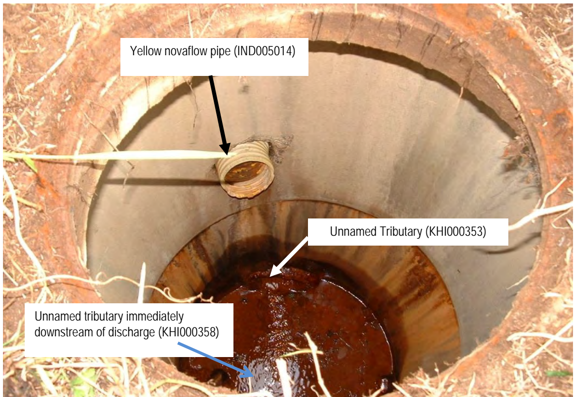
Photo 1 The view down manhole 2
