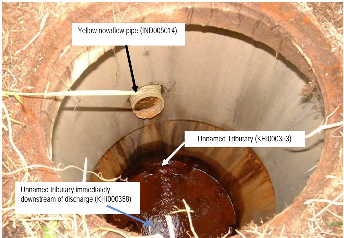
Photo 1 The view down manhole 1 2
