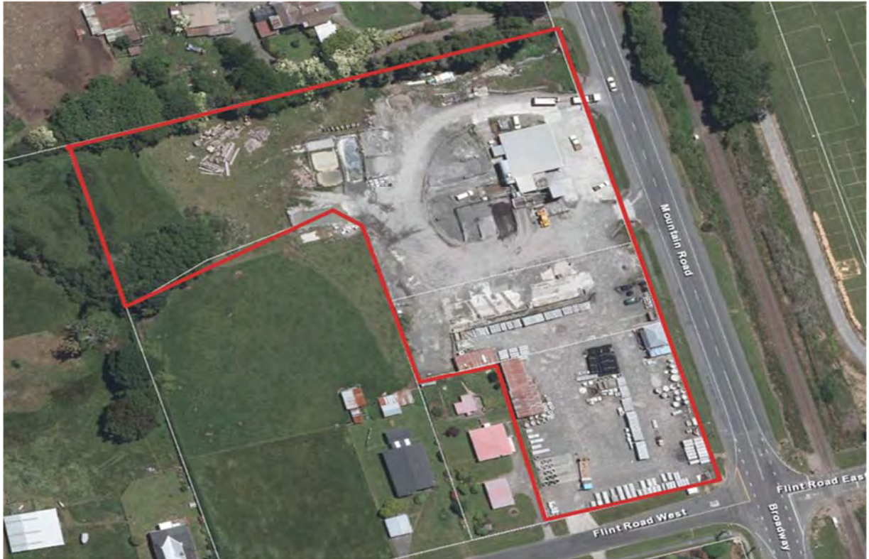
Figure 4 Location of the Fletcher Concrete site (Firth Industries and Humes Pipeline Systems), Stratford
