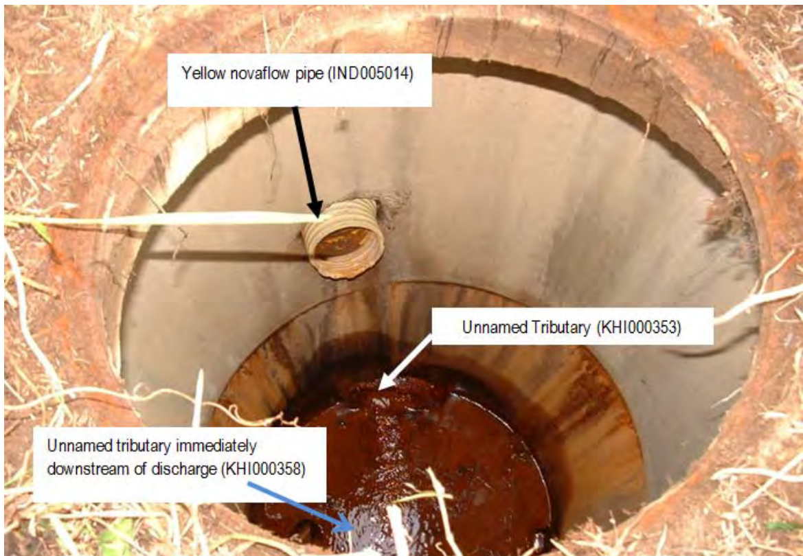
Photo 1 The view down manhole 1
