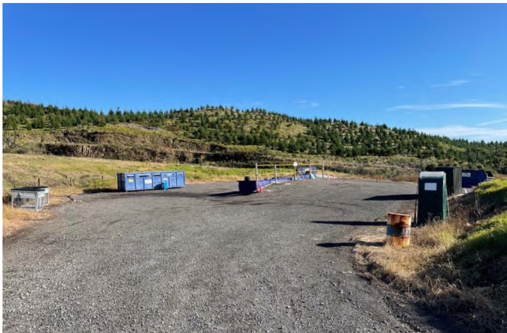
Photo 1 Inglewood landfill transfer station
