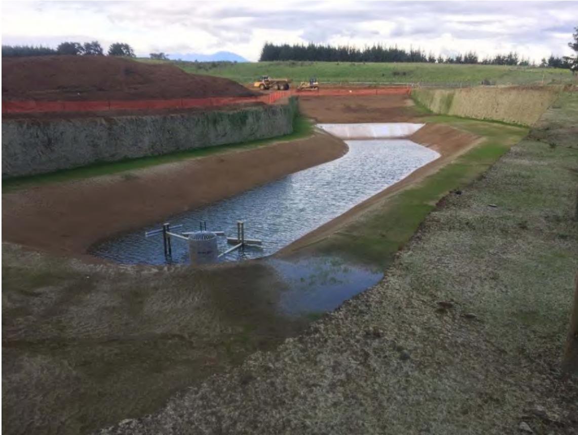
Photo 2 Borrow area sediment pond, November 2020
