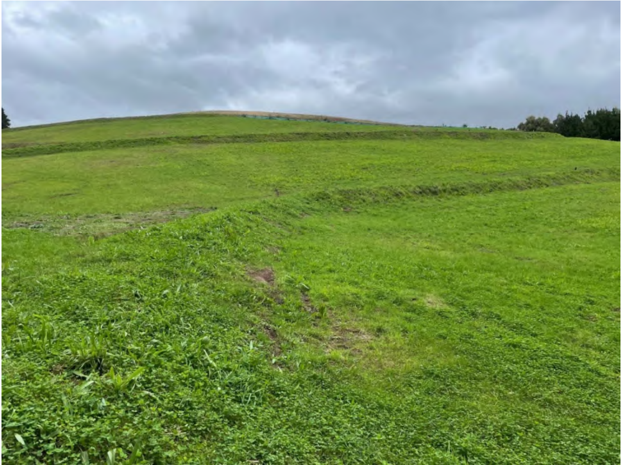
Photo 1 Stabilised northern toe of Stage 3, May 2022
