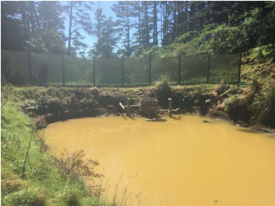
Photo 5 Floating decant system in the large silt pond, March 2021
