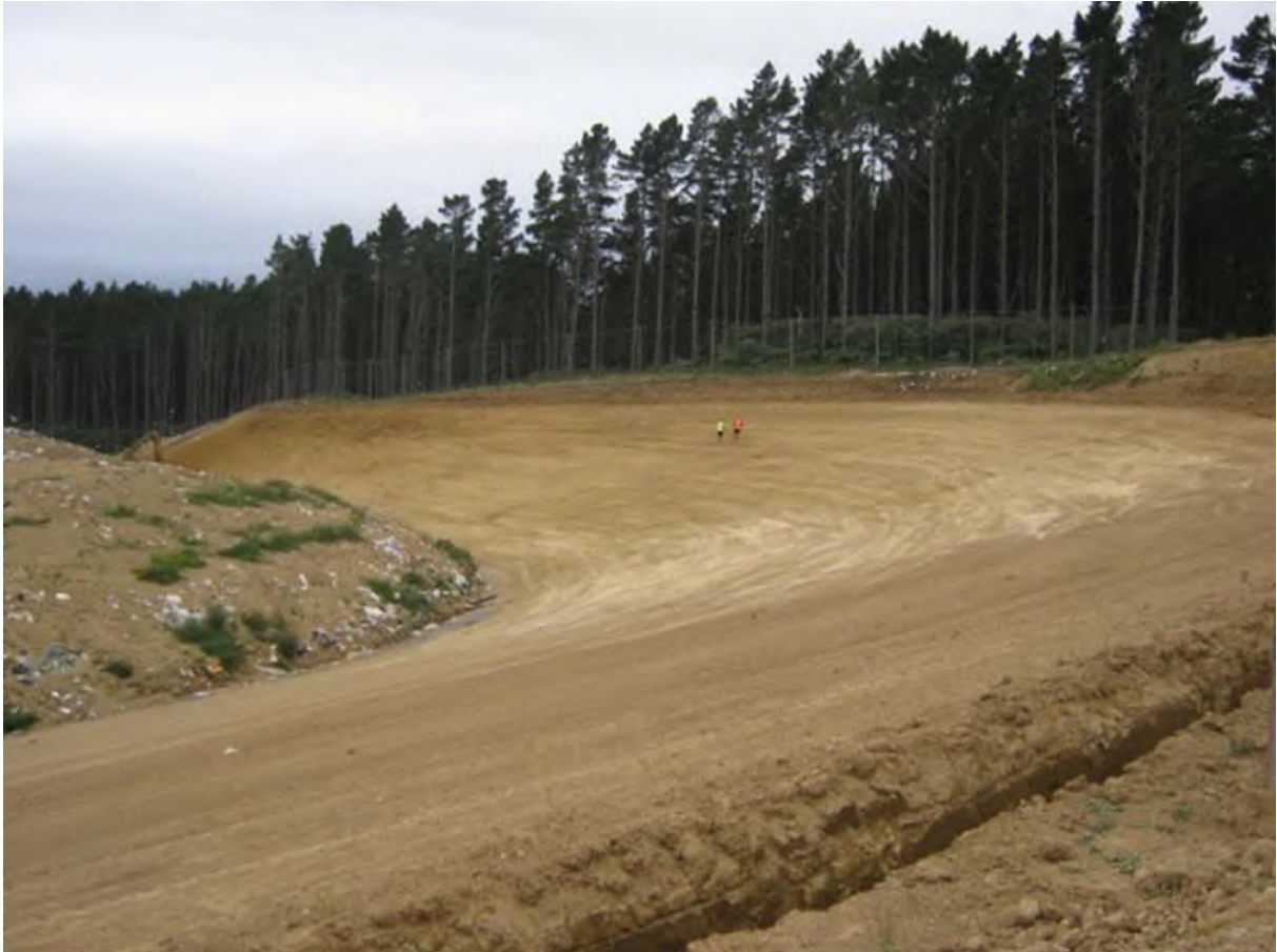
Photo 6 Stage 3 extension works, February 2011
