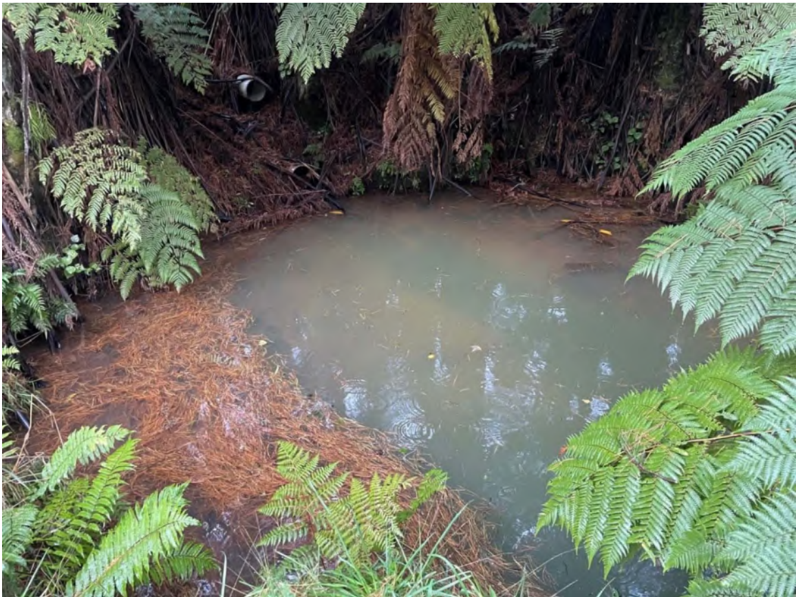
Photo 10 Western small silt pond, 15 June 2022
