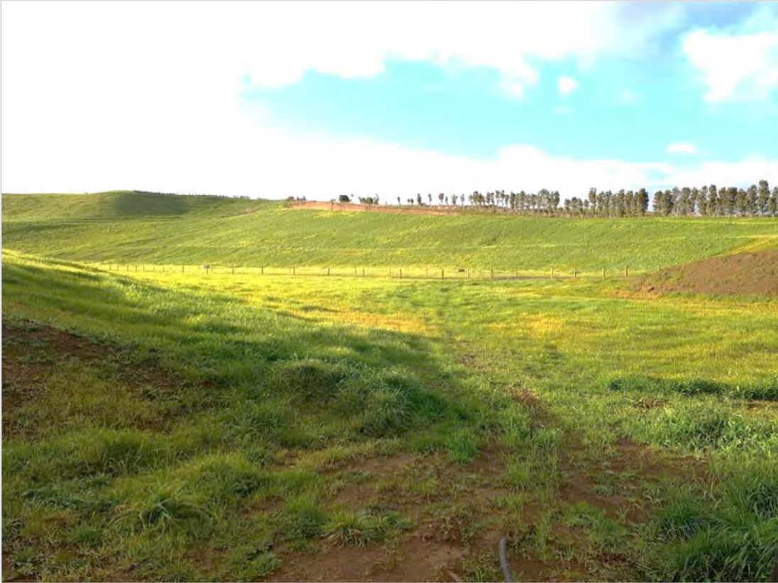
Photo 6 Central Landfill, 12 June 2019 – southern side of southern gully after stabilisation
