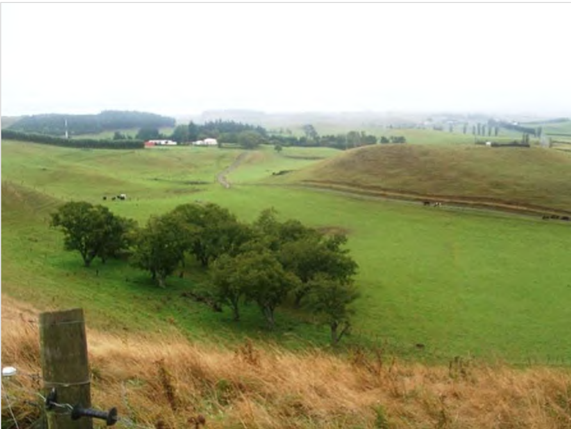
Photo 3 Central landfill site (south westerly view from the east side of the site)
