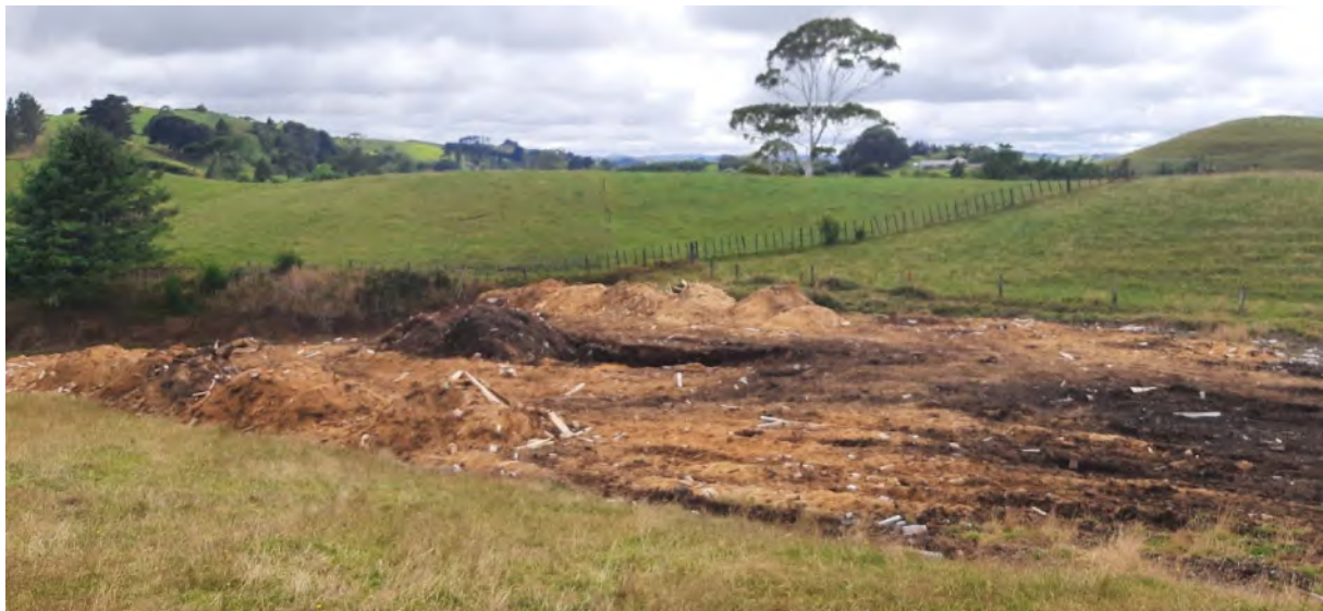
Photo 2 Value Timber Ltd site inspection 26/01/2022
