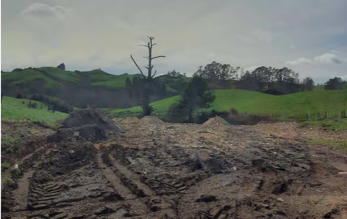
Photo 3 Value Timber Ltd site inspection 20/06/2022
