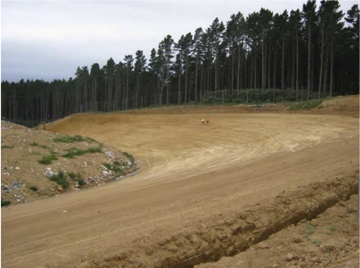
Photo 4 Stage 3 extension works, February 2011
