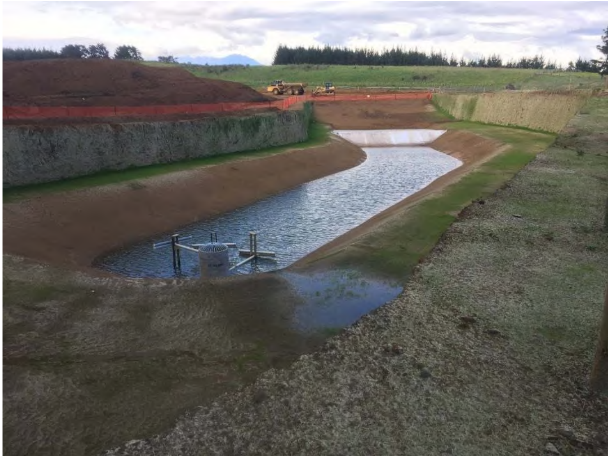
Photo 7 Borrow area sediment pond, November 2020
