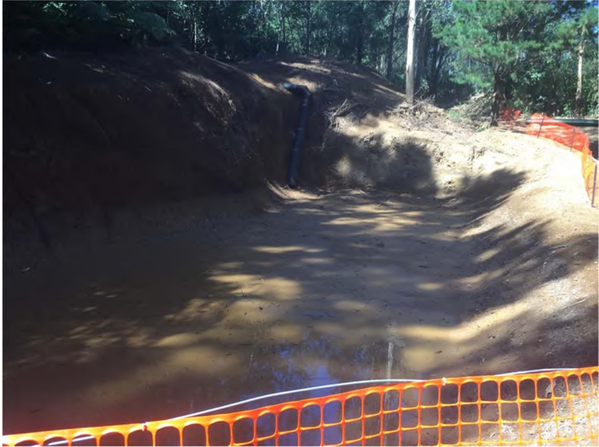
Figure 8 Completed fore bay to large silt pond, March 2021
