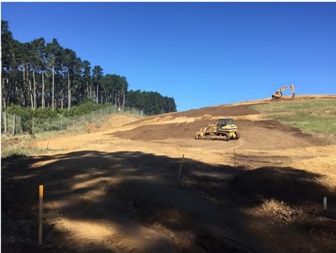
Photo 2 Application of top soil on north-eastern batter of Stage 3, April 2021
