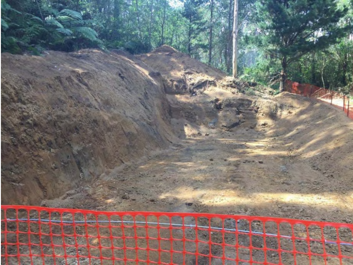
Photo 11 Fore bay being constructed for the large silt pond, February 2021
