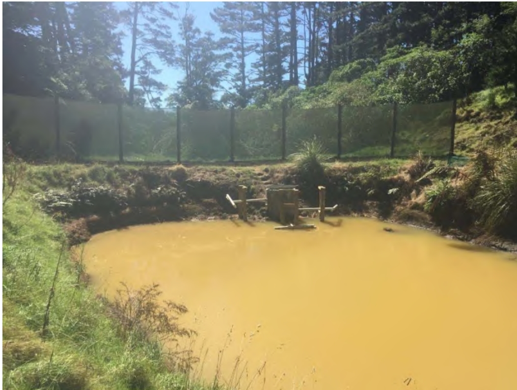
Photo 12 New floating decant system in the large silt pond, March 2021
