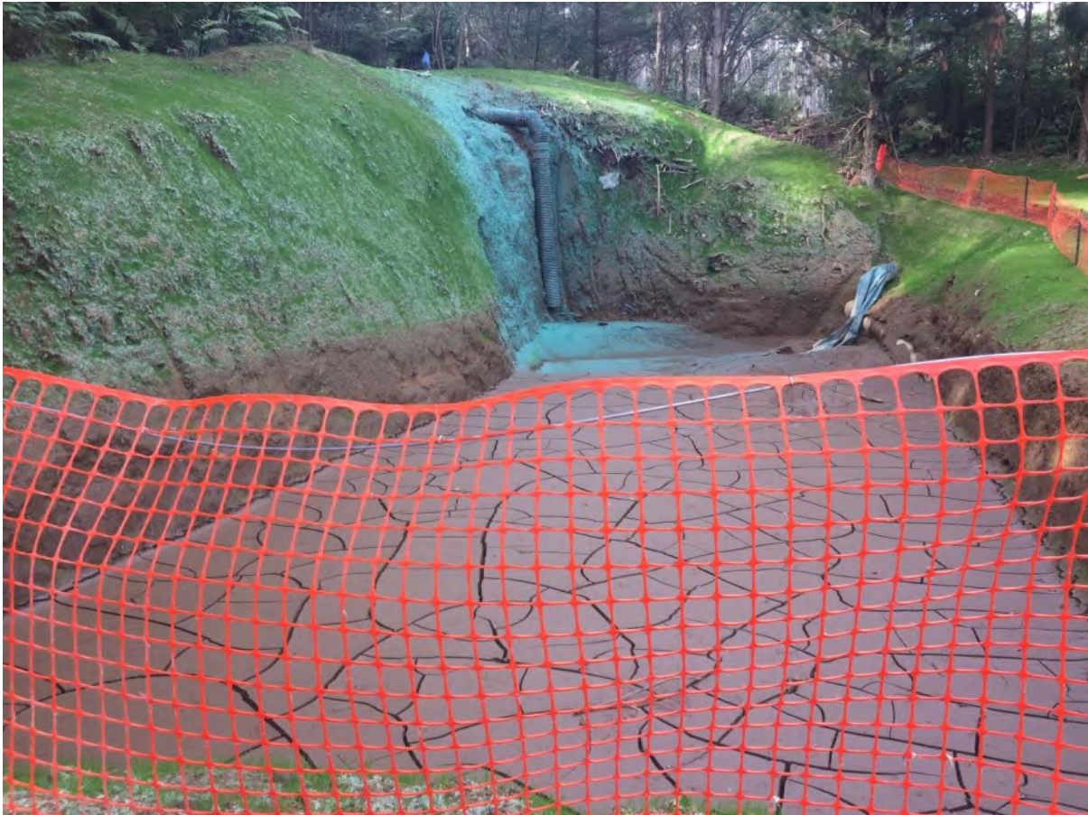
Photo 3 Pretreatment pond for large silt pond, May 2021
