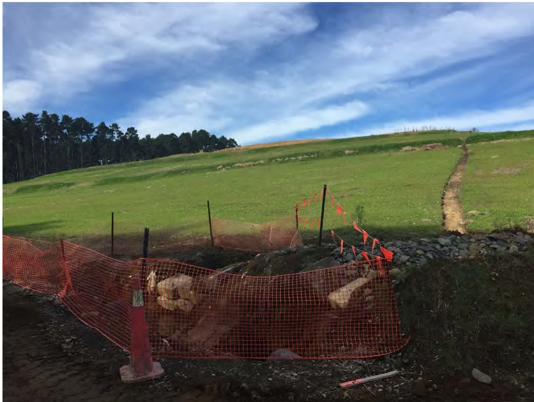
Photo 14 Northern face of the landfill, May 2021
