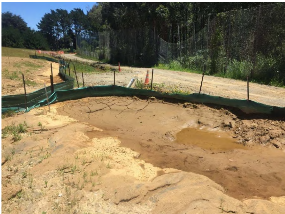
Photo 8 Silt fence, December 2020
