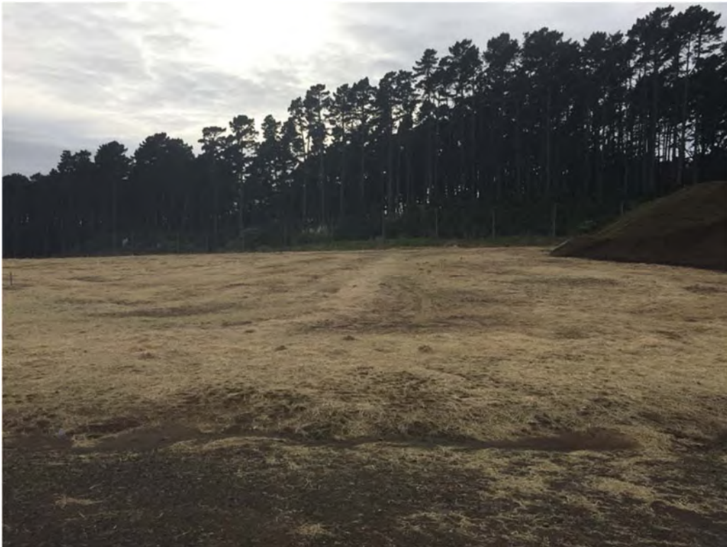
Photo 15 Stabilisation on southern end of the landfill, June 2021
