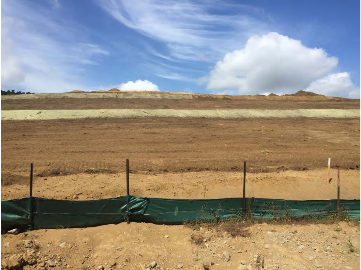
Photo 10 Hydroseeded bunds on northern face of the landfill, February 2021
