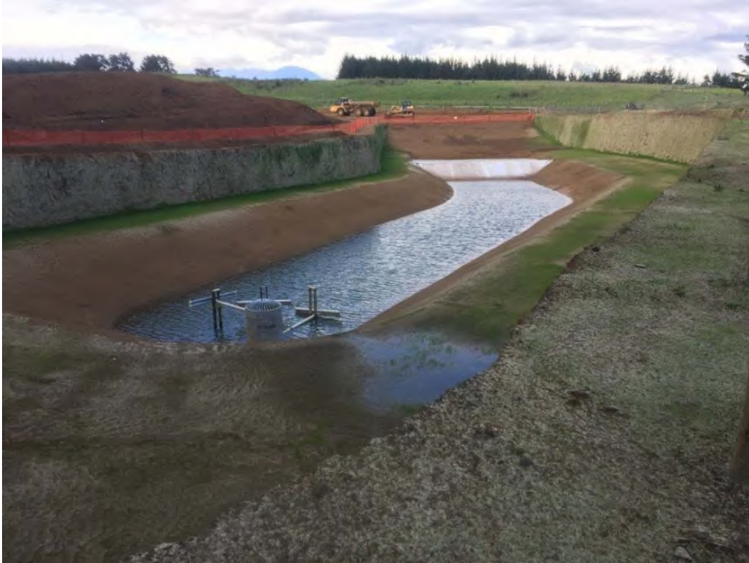
Photo 3 Borrow area sediment pond, November 2020
