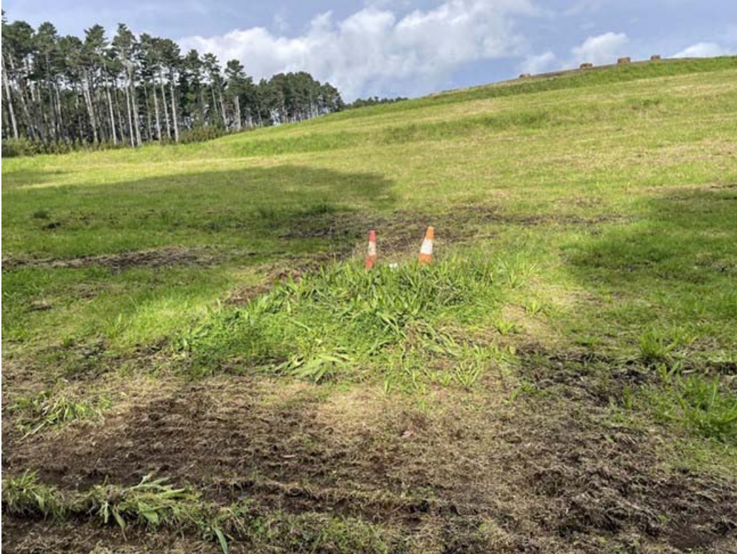
Photo 1 Stabilised northern toe of Stage 3, May 2023
