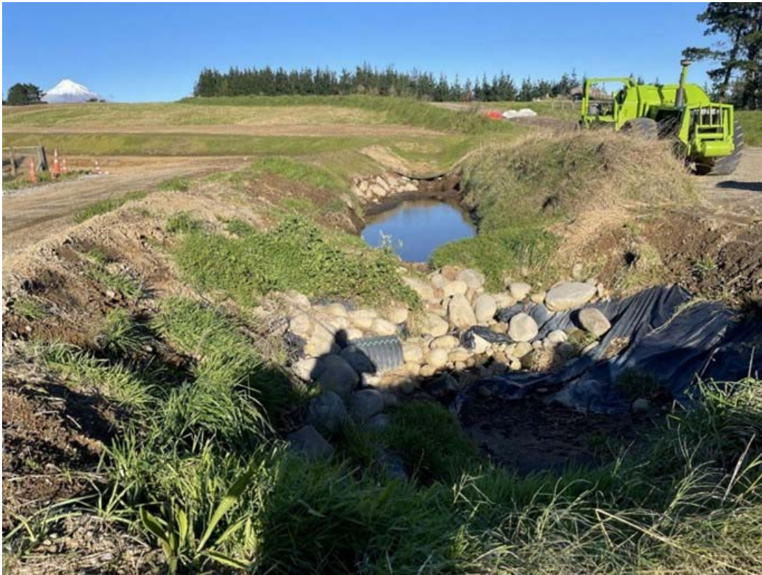
Photo 4 Amended drainage and access during capping works for Stage 2 remediation, June 2023
