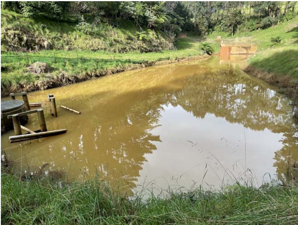
Photo 6 Floating decant system in the large silt pond, May 2023
