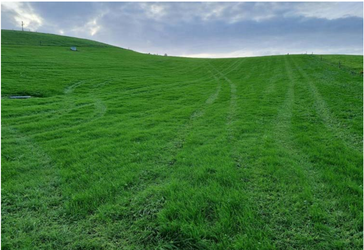
Photo 4 Batter at the toe of the fill area, June 2024
