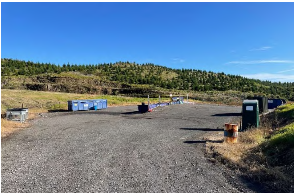
Photo 1 Inglewood landfill transfer station
