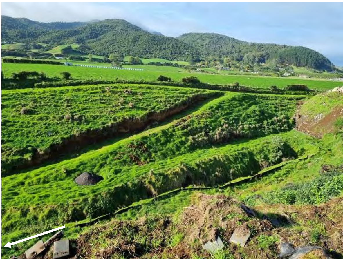
Photo 5 Bishop cleanfill. The silt retention fence required extension in the direction indicated by the arrow, 27 May 2024
