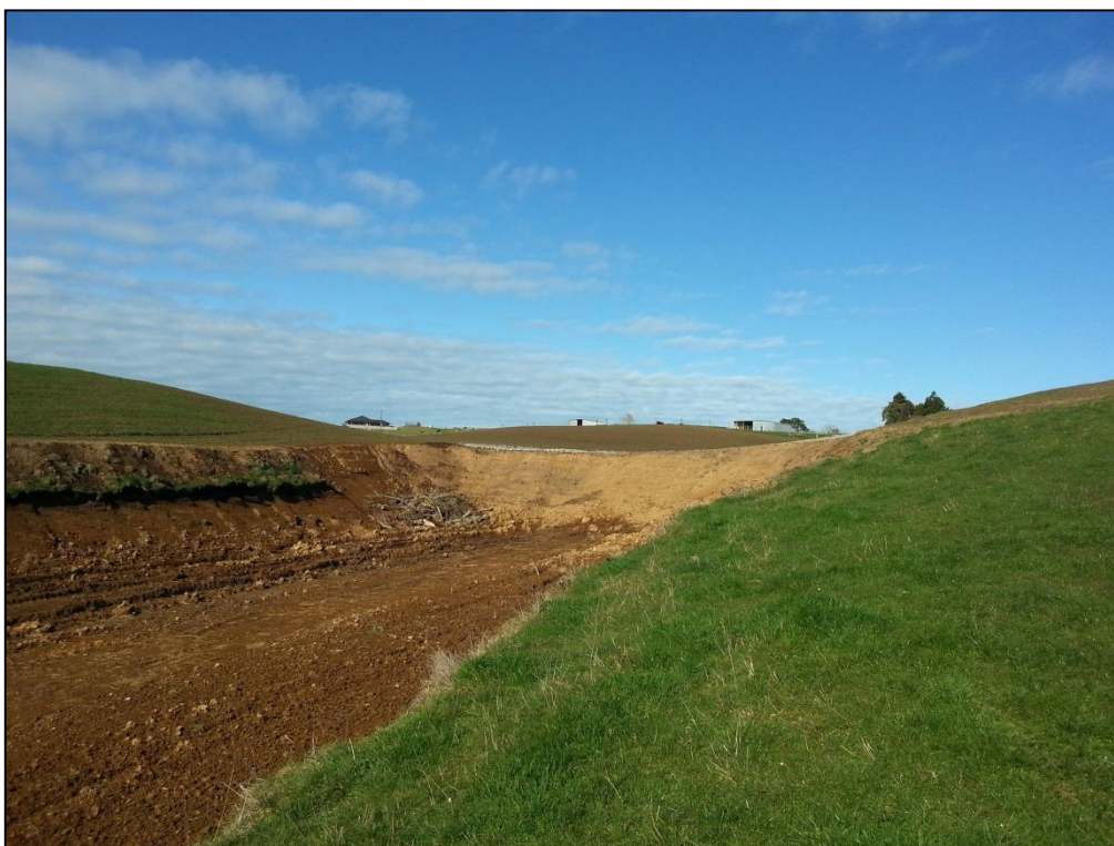
Photo 1 Newly prepared fill area after reinstatement of stage 1
