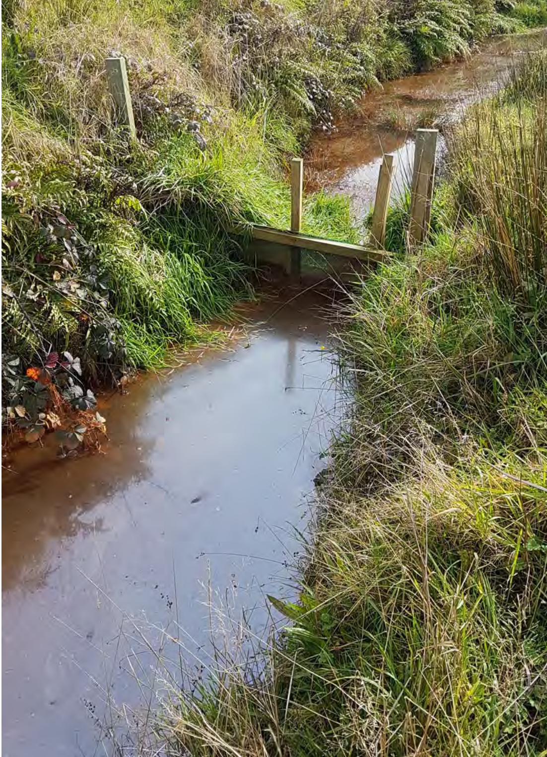
Photo 1 Upgraded in-drain silt control fence
