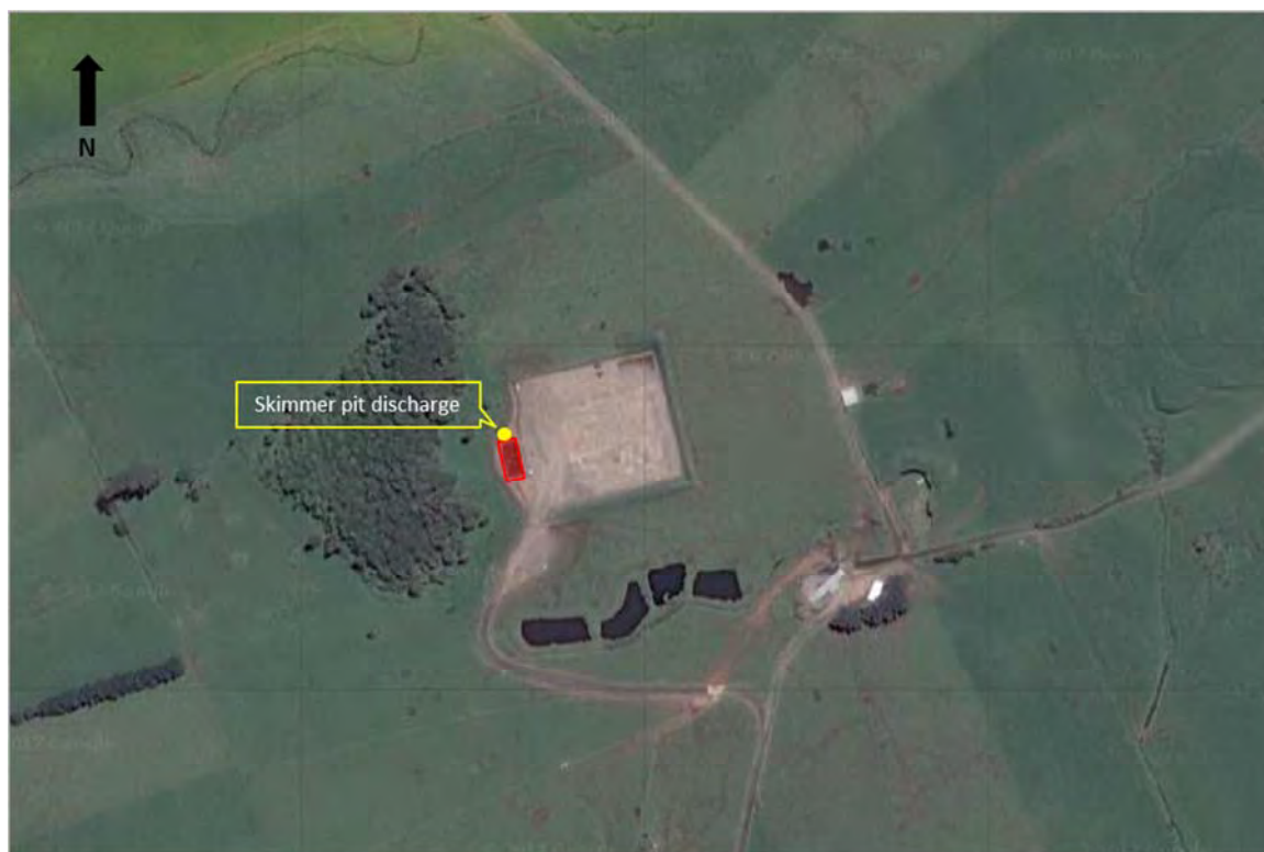
Figure 1 Aerial view showing location of skimmer pits (red) and discharge point (yellow)
