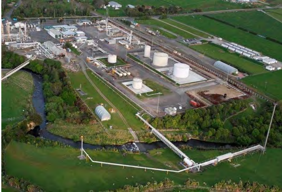
Photo 1 Kapuni Production Station
