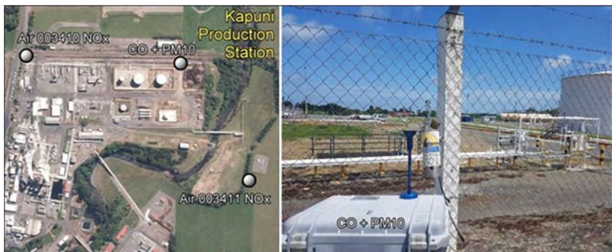
Figure 2 Air monitoring sites at Kapuni Production Station for 2018-2019
