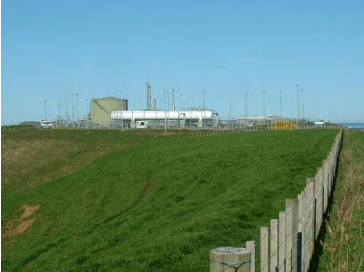
Photo 1 Rimu Production Station
