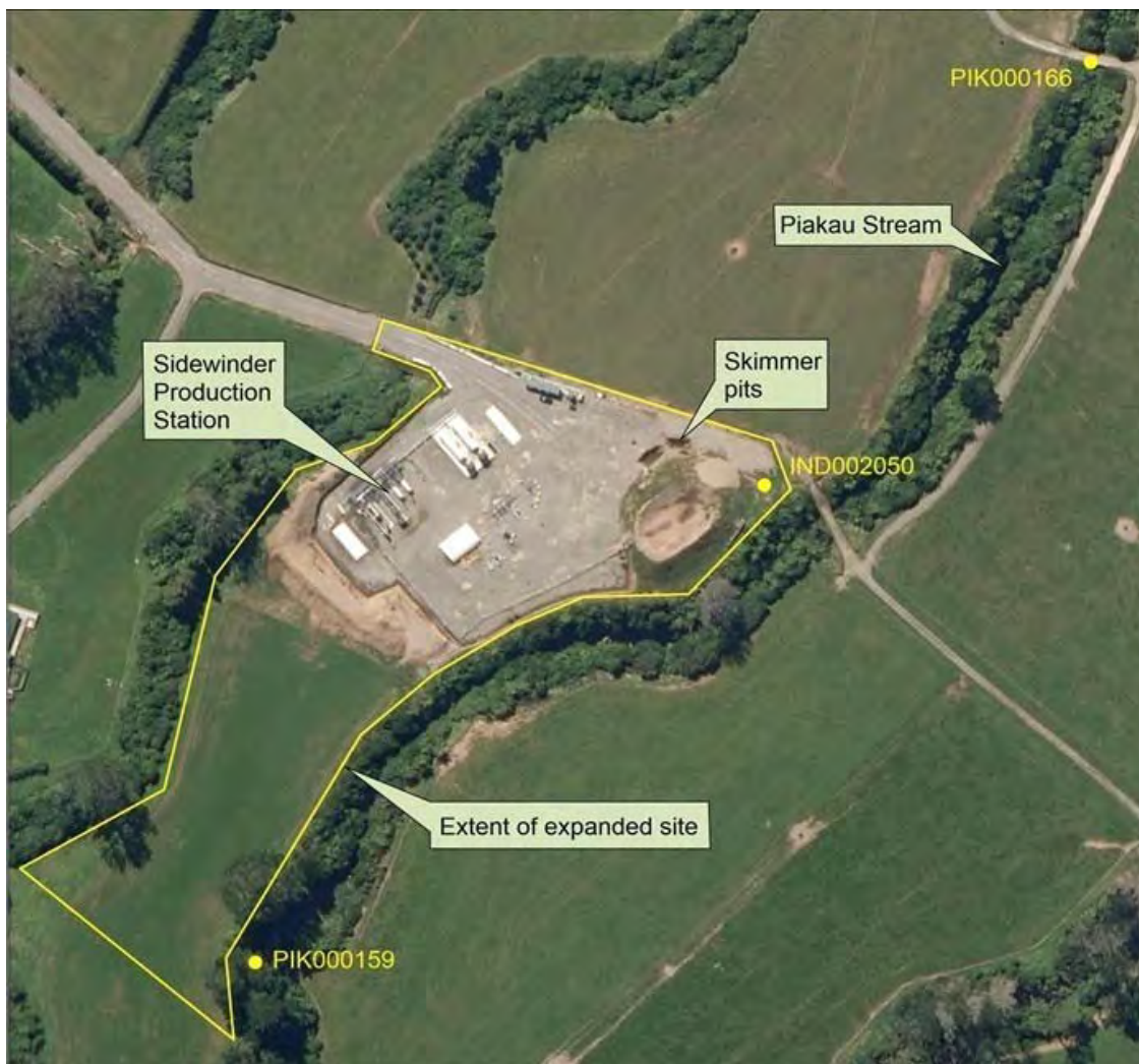
Figure 1 Sidewinder Production Station and associated water quality sampling sites
