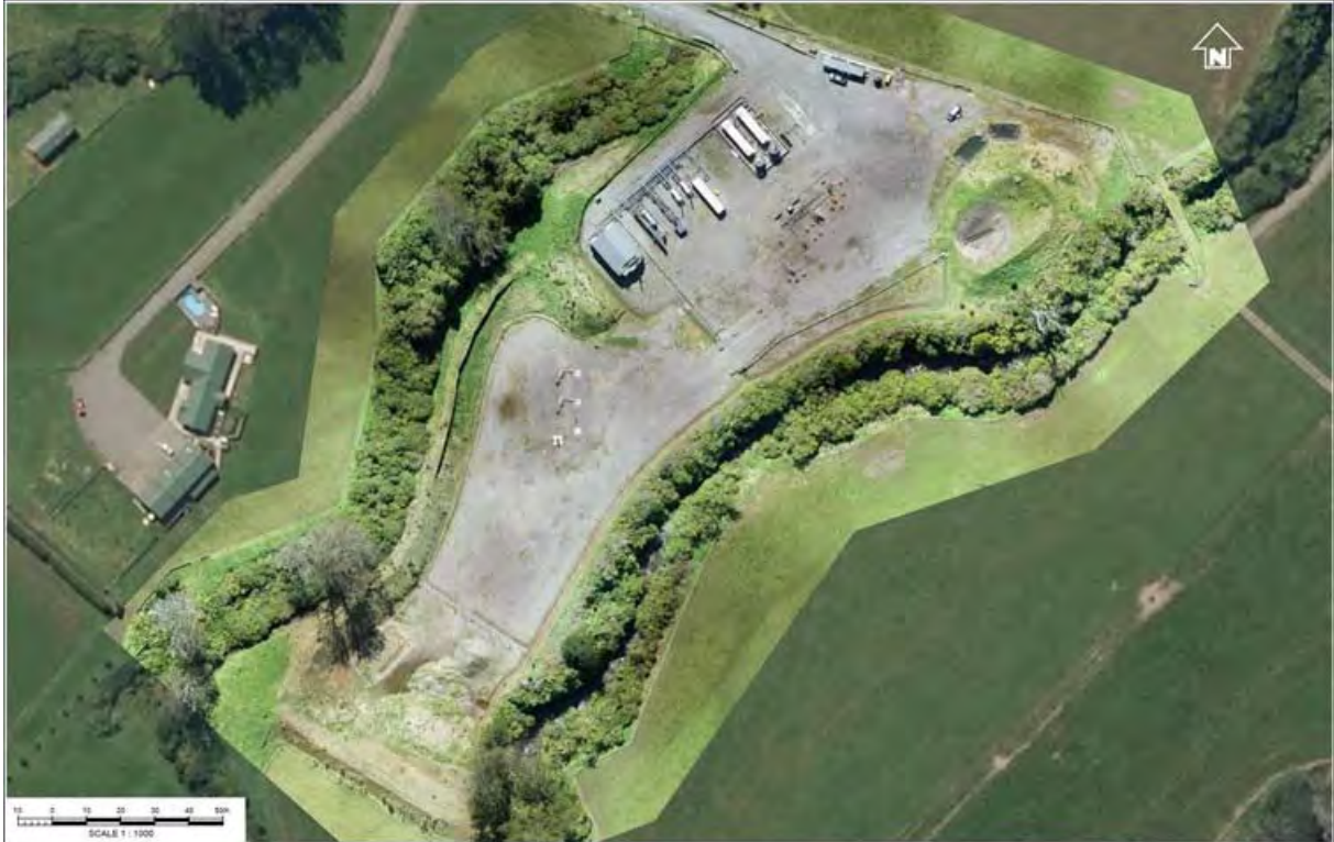
Photo 1 Sidewinder Production Station and wellsite (2019)
