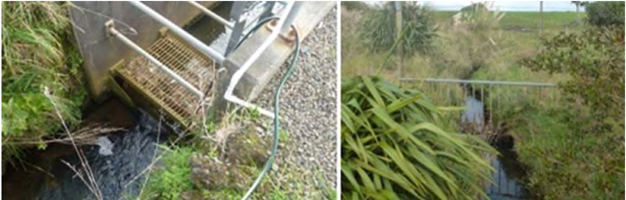
Photo 2 Discharge to the Ngapirau Stream
