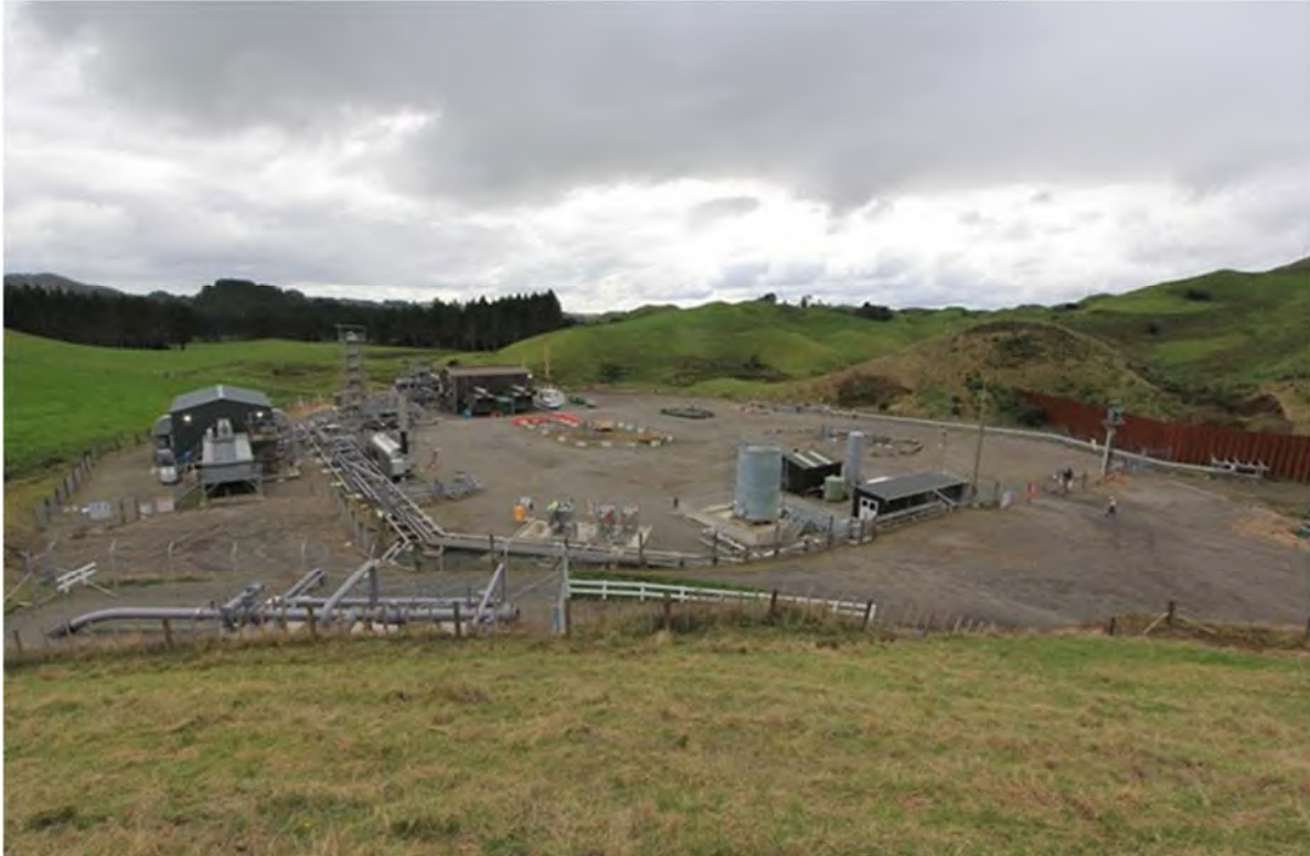
Photo 1 Ahuroa B gas storage facility layout facing North West May 2014
