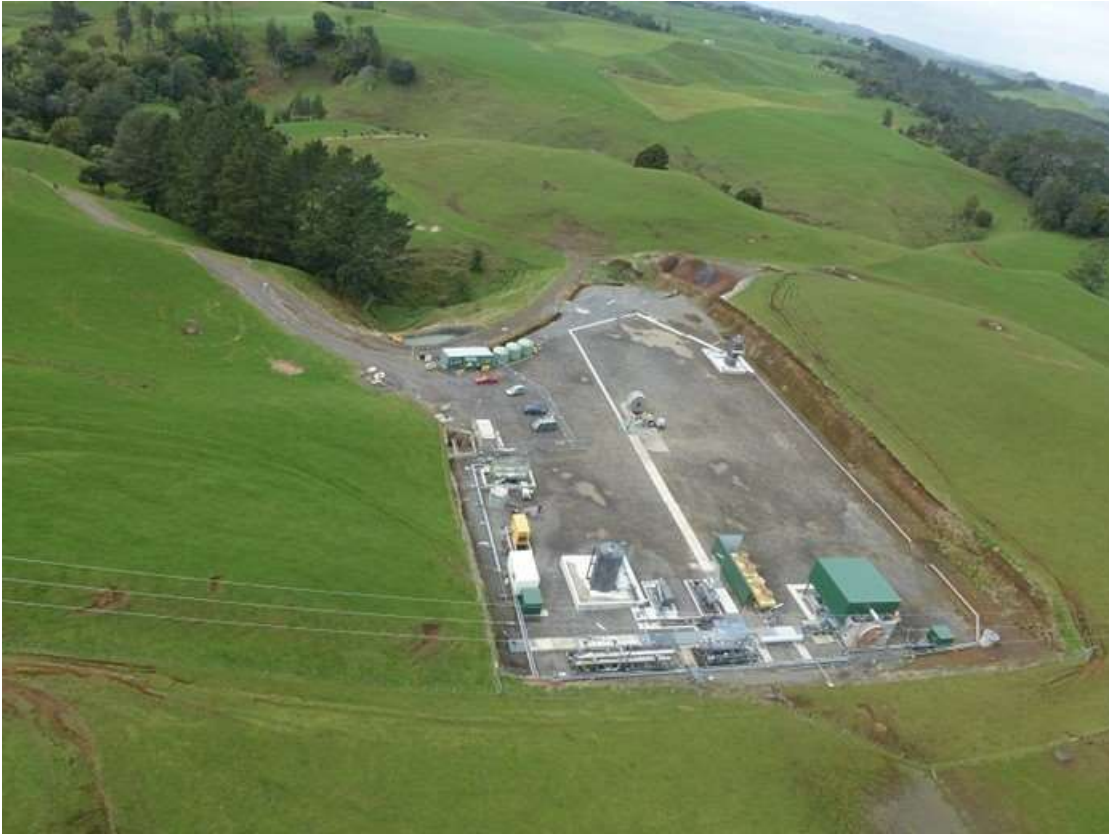
Photo 2 Kowhai-A Production Station
