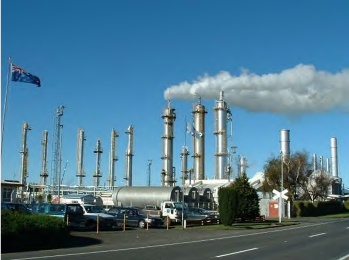
Photo 1 Kapuni Gas Treatment Plant (KGTP) during three train operation
